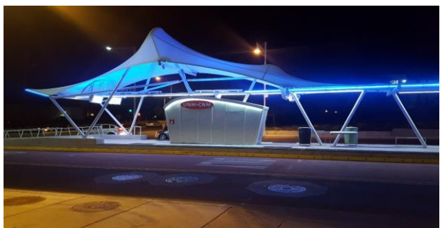
Example of an ART transit platform
