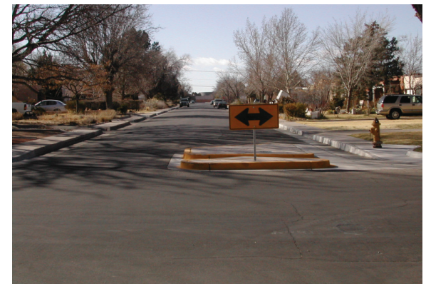
A diverter in the Highland area prevents through-traffic on heavily impacted residential streets
