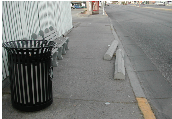
Obstacles in sidewalks can make passage difficult, particularly for wheelchair users
