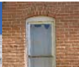
Segmented brick arch over double-hung window
