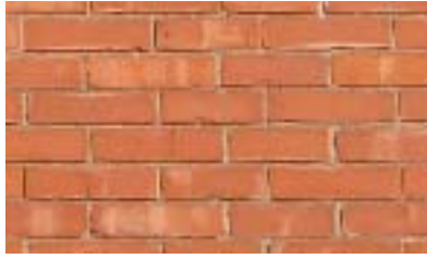
Hard bricks were available after 1899.
