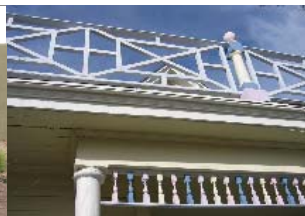
Balustrade at roof
