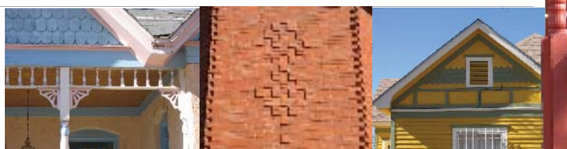
Spindlework and jigsaw-cut trim on porch
