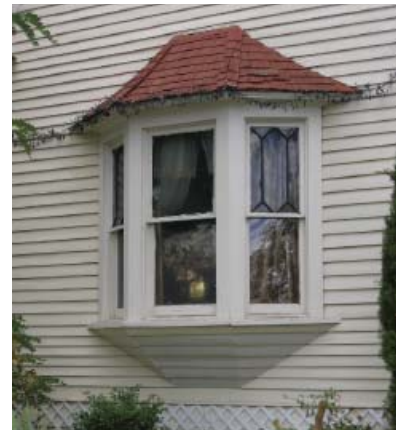
Oriel: Project from the side of a building, like a bay window, but are supported by brackets.
