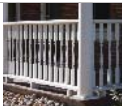
Spindles at porch railing
