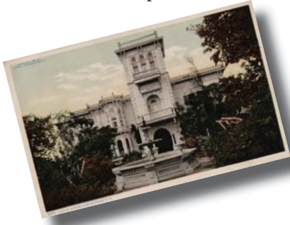
Attached tower elements are common as exemplified by the now demolished Huning Castle.
