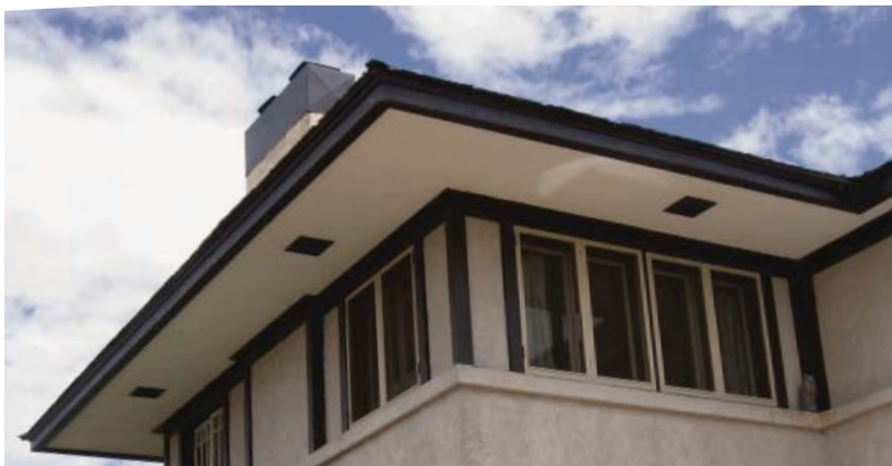
Ribbon: Three or more contiguous windows. Common for Bungalow (craftsman) and Prairie styles. All post-1900 eclectic styles may include ribbon windows, but not typically on the front.
