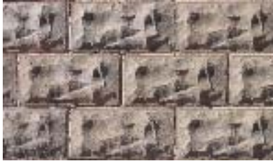
Before concrete blocks were available locally, molds could be purchased to make cast stone.
