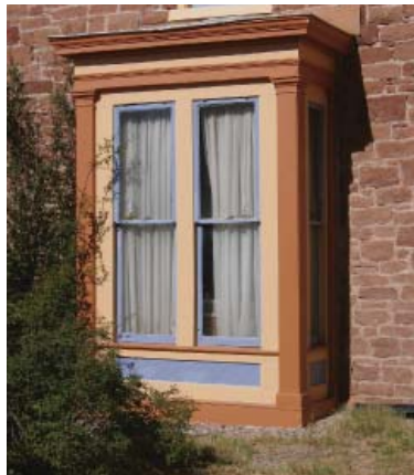
Box Bay: Project from the side of a house with 90 degree angles at the corners.
