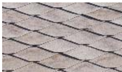
Asphalt shingles - This pattern was known as the "French method".
