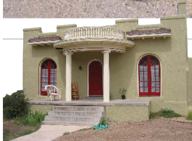
Neoclassical porch with balustrade
