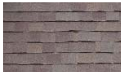
Asphalt shingles
