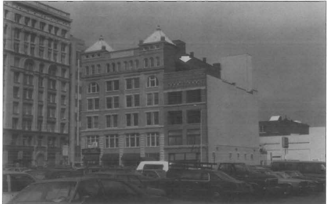
Left: This rooftop addition has substantially altered the historic profile and proportions of a three-story row house; more important, it has interrupted the uniform roof height of the block. The greenhouse is also a jarring element in an otherwise intact 19th century streetscape. Below: A sizeable employee lounge was added atop this four-story historic commercial building. Because the rooftop addition has been set back from both the front and side roof edges against a party wall, the historic character of the building and the district have been preserved.
