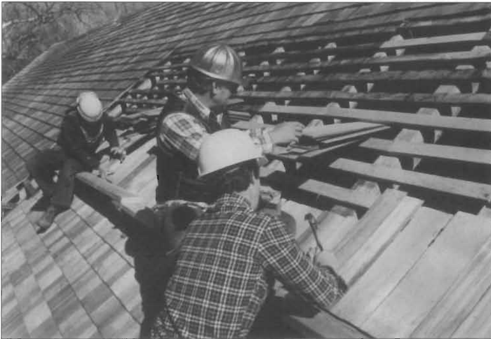
The size, shape, and detailing of the historic shingles as well as the method of fabrication and installation were carefully researched prior to selecting this new wood-shingle roofing.
