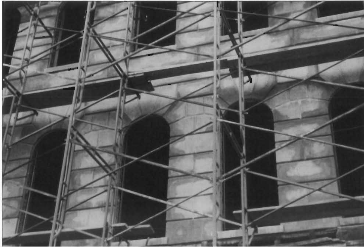
Composite patching with a cementitious mixture is being used to repair eroded areas of this sandstone facade.
