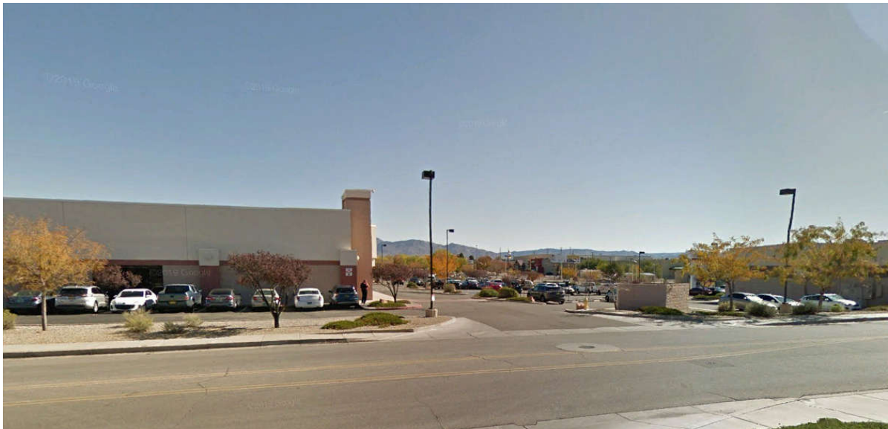
Figure 5: Subject Site Developed Land (East View)
