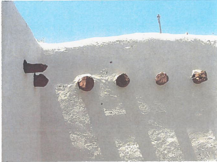
Figure 32 Typical Cement Stucco Walls
