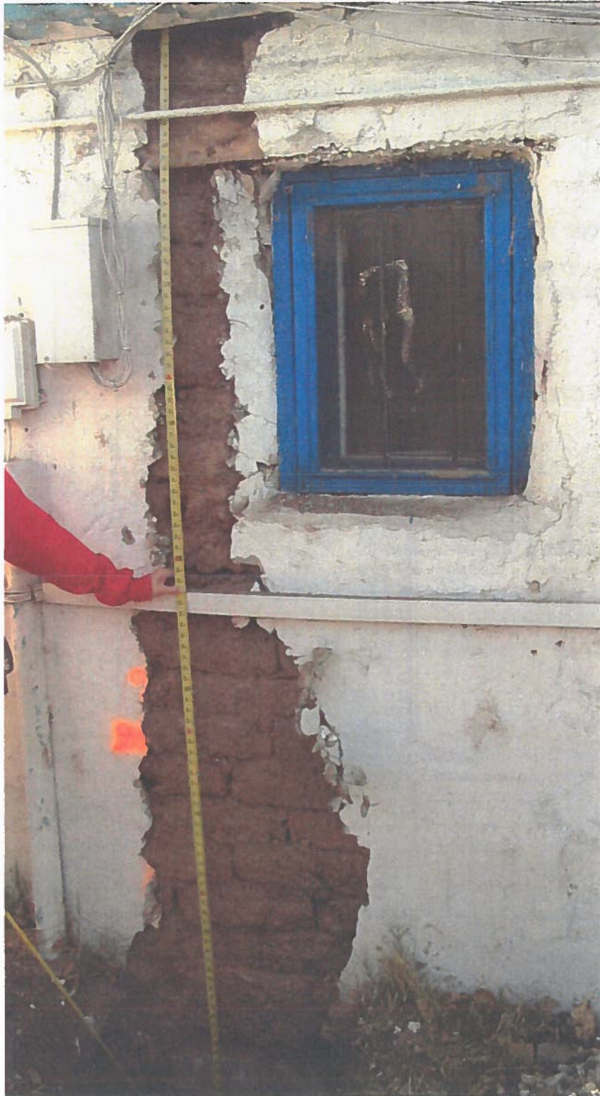
Figure 35 Typical Adobe Wall Construction
