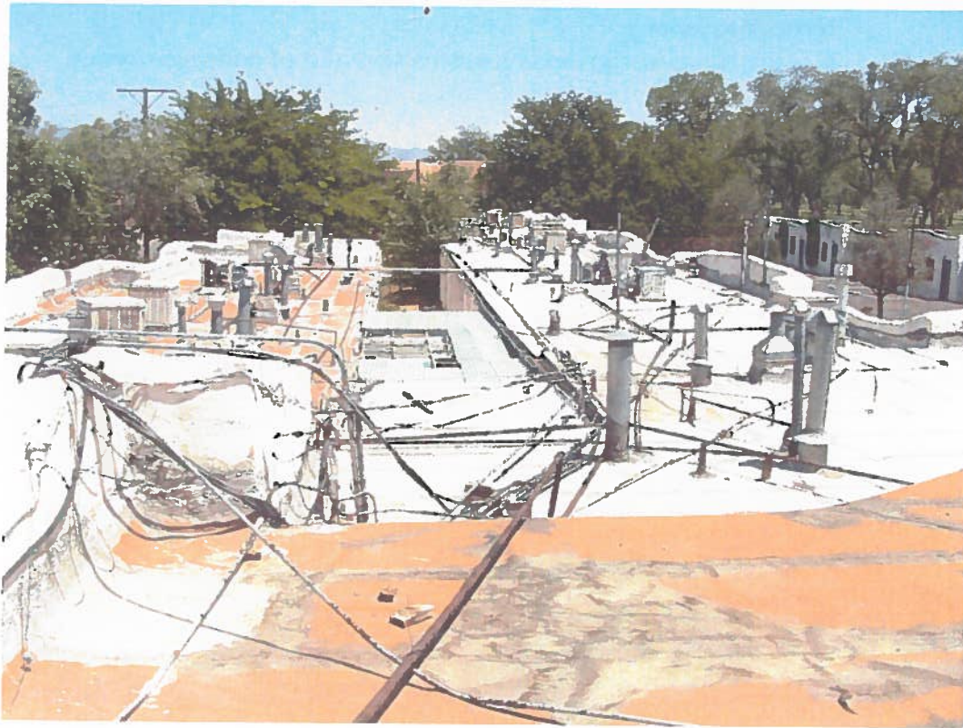
Figure 41– Roofing Materials at Building 1.
