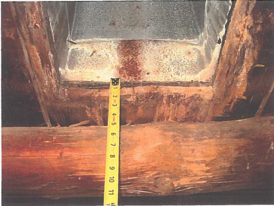
Figure 23 Roof Sheathing and Layered Roofing Sheets
