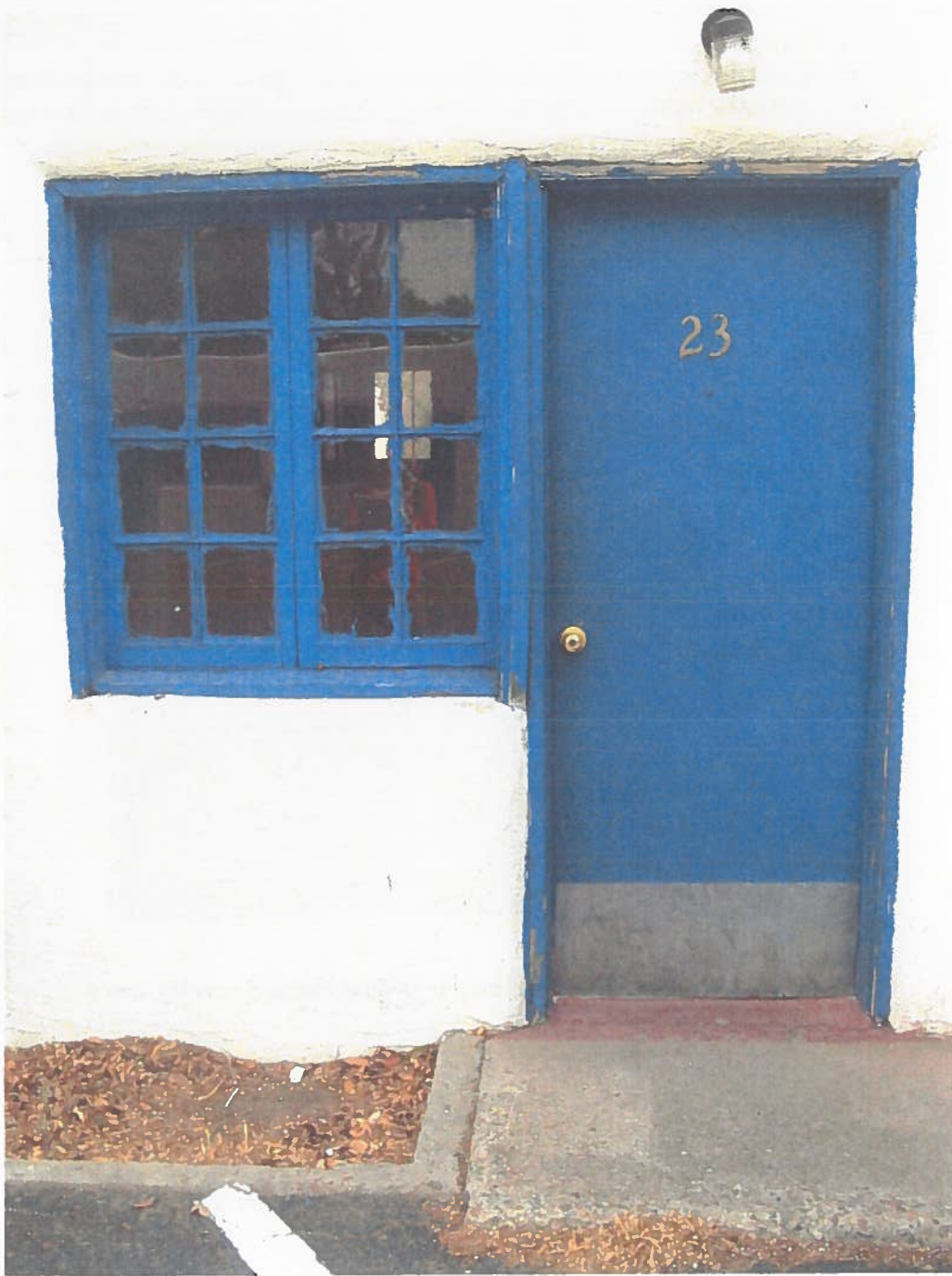
Figure 46 - Multi-pane Window and Typical Wood Exterior Door
