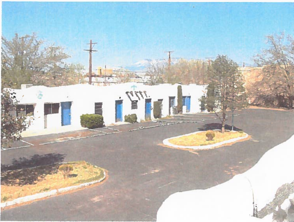
Figure 10 Asphalt Paving and Landscape Island
