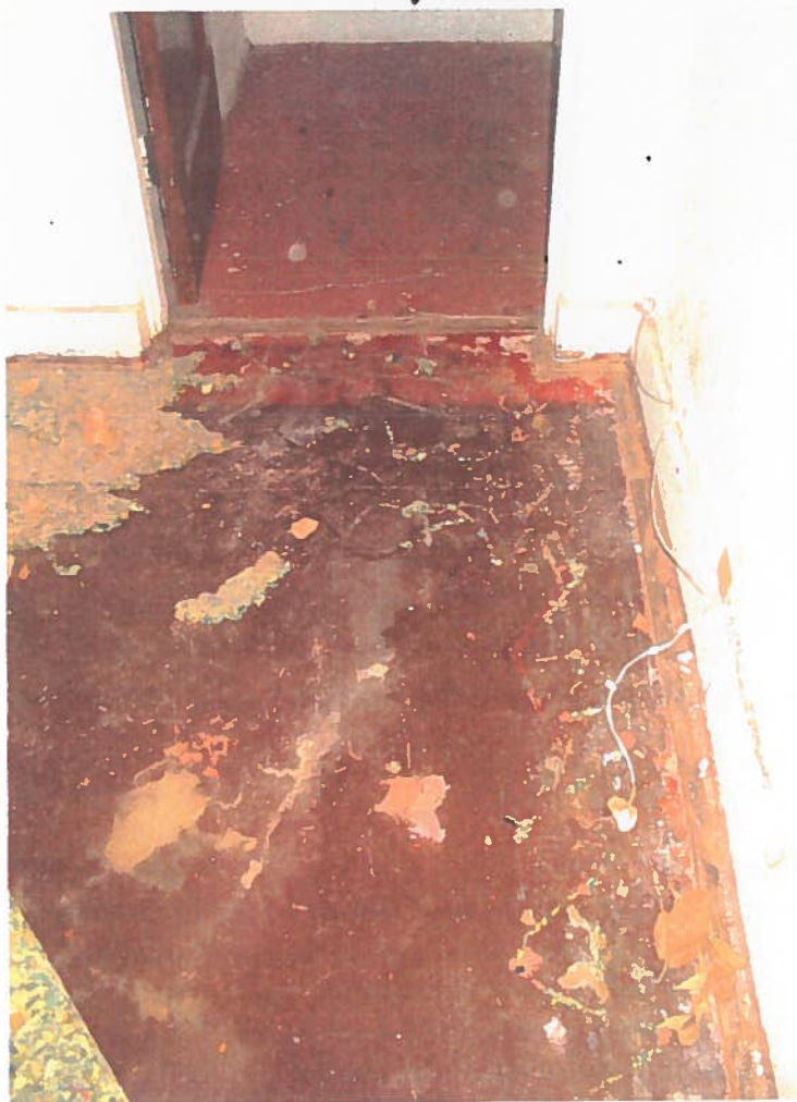
Figure 20 Cast in Place Concrete Floor Slab
