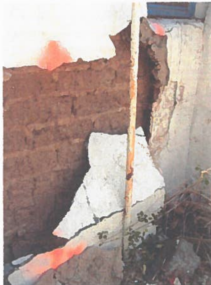
Figure 37 Cement Stucco at North East Adobe Wall
