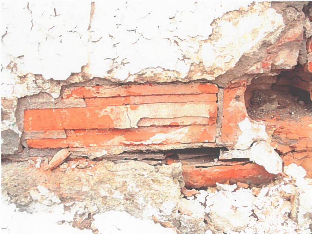
Figure 30 Hollow Clay Tile Unit
