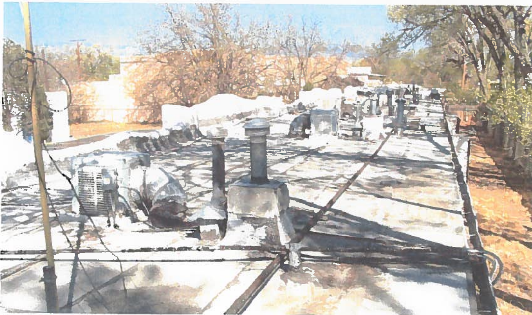
Figure 29 Roof Penetrations at South Room Block
