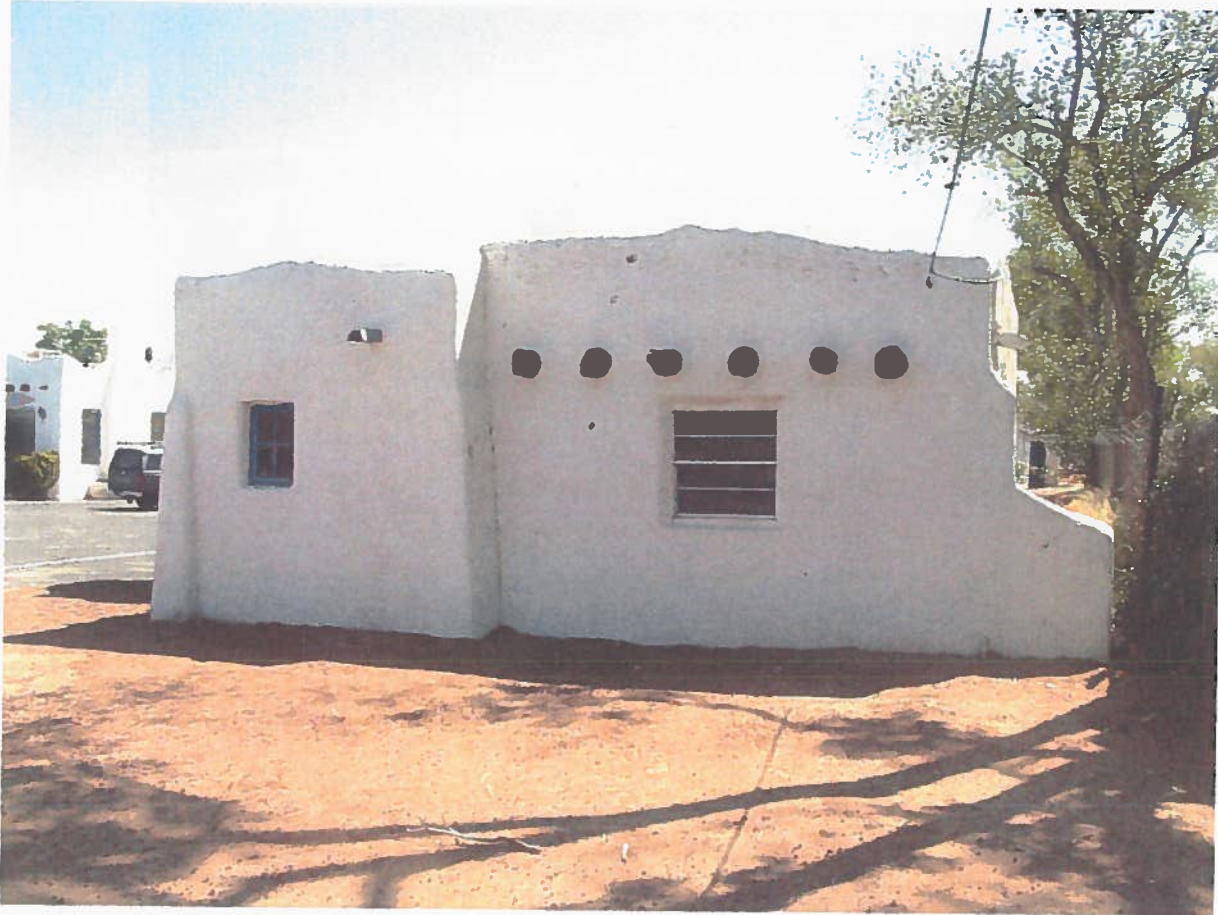
Figure 31 South West Rooms Built of Hollow Clay Tile
