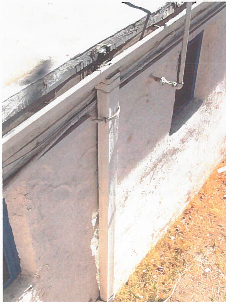
Figure 42 Gutter and Downspout Assembly
