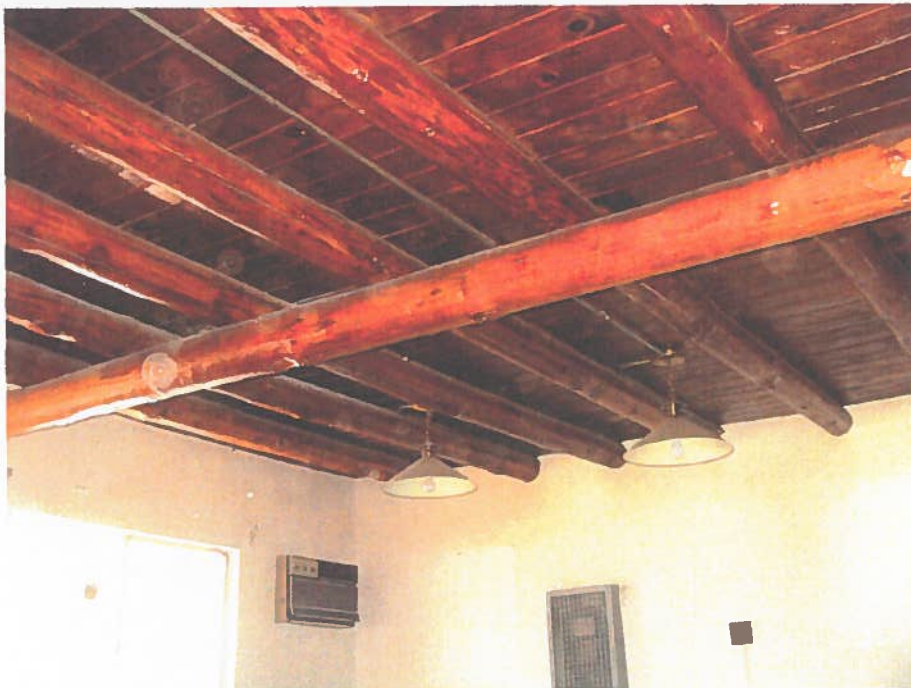
Figure 24 Roof Vigas With Mid-Span Support Viga
