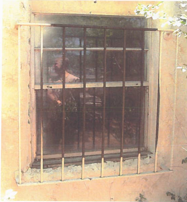
Figure 45 - Single Hung Window With Security Bars
