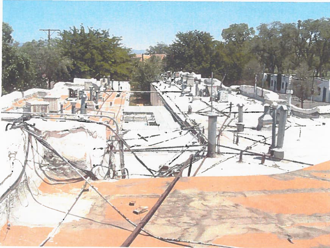
Figure 28 Roof Penetrations at North Room Block
