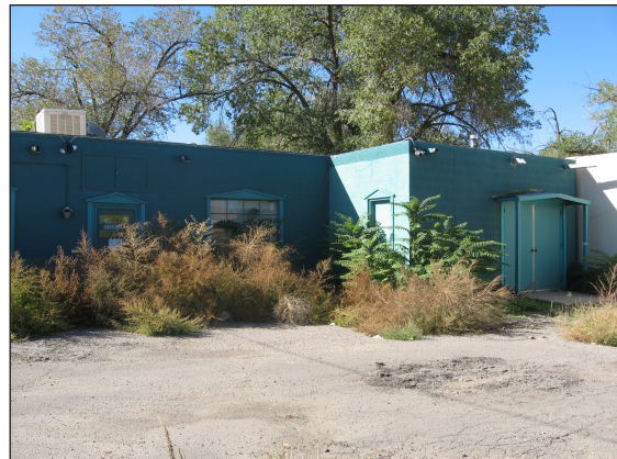
Distressed property along Mountain Road, west of 12th Street
