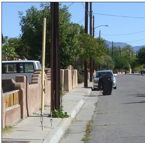
Utility poles and guy wires obstructing the public sidewalk
