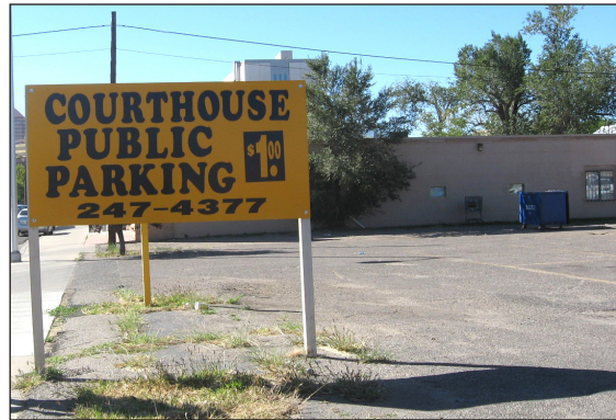
Non-conforming commercial parking lot along Fourth Street
