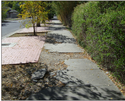
Deteriorated sidewalk
