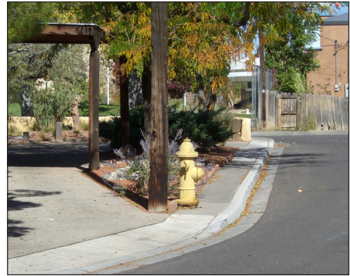
Fire hydrant obstructing very narrow sidewalk
