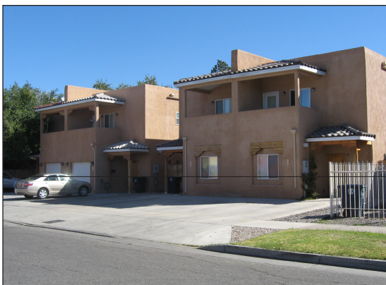
Townhomes along 11th Street with no area left for landscaping in the front setback
