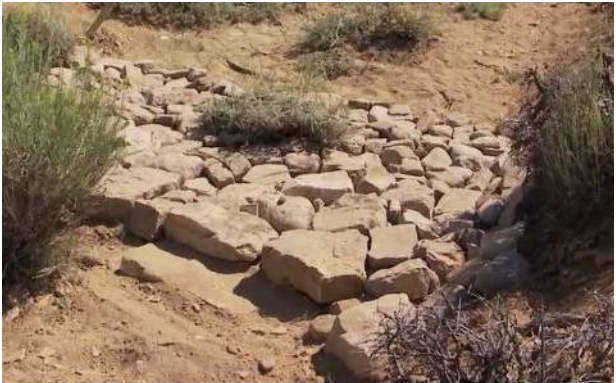
One Rock Dam
