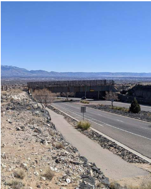
Land bridge across Paseo del Norte
