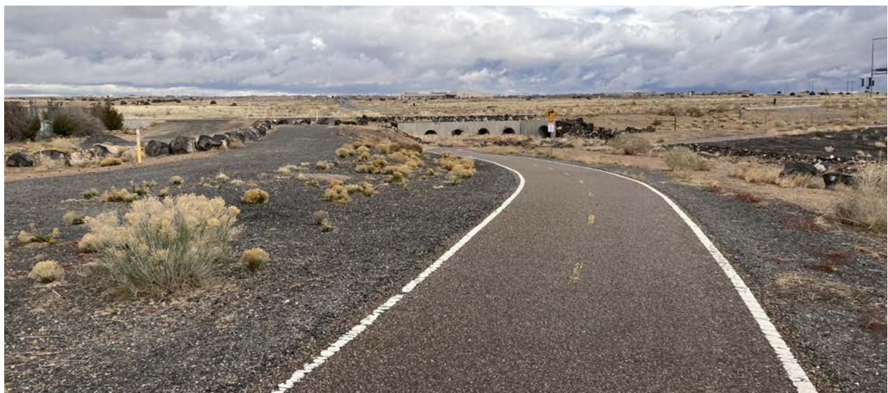
Resource management requires coordination with multiple agencies for a variety of assets like the Boca Negra Dam Trail (above).
