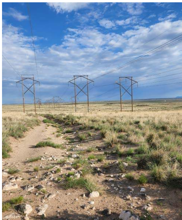
Existing PNM easement roadway
