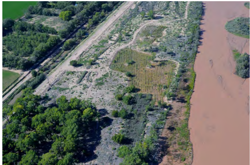
Inundation of the Middle Rio Grande Restoration Project at Sites 5D and 5E, September 2013
