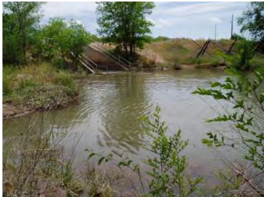
Central Outfall Wasteway
