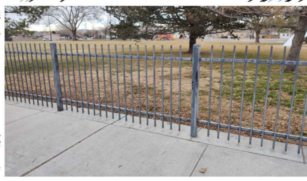
TUBULAR STEEL FENCE BASIS OF DESIGN (EXISTING)
