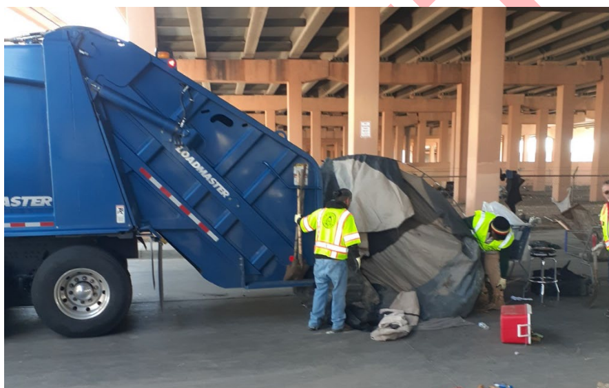
Photo 3.6e – SWD Tent Demolition 3/29/2024
