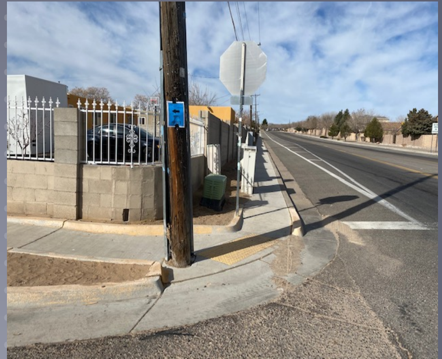
Utilities located within the Curb Access Ramps
