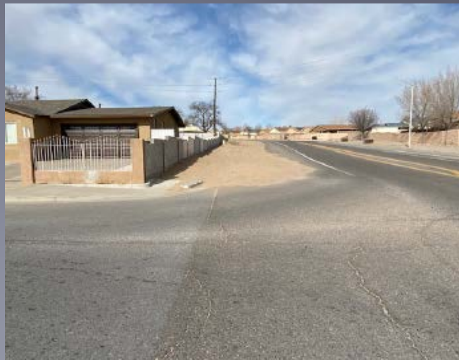
Lack of Sidewalk, Curb, Gutter, Storm Drainage Infrastructure and Bicycle Facilities on the south side of Devargas Road.
