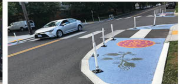
Portland, OR Painted Curb Extension source: bikeportland.org
