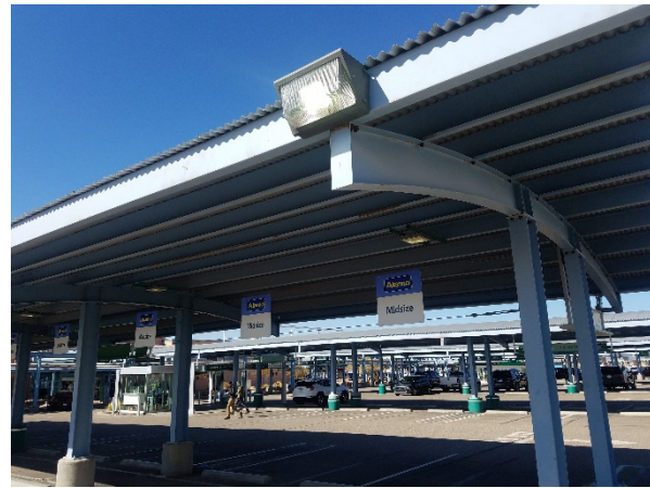
Figure 1: Existing Canopy in Mid-Eastern Block
