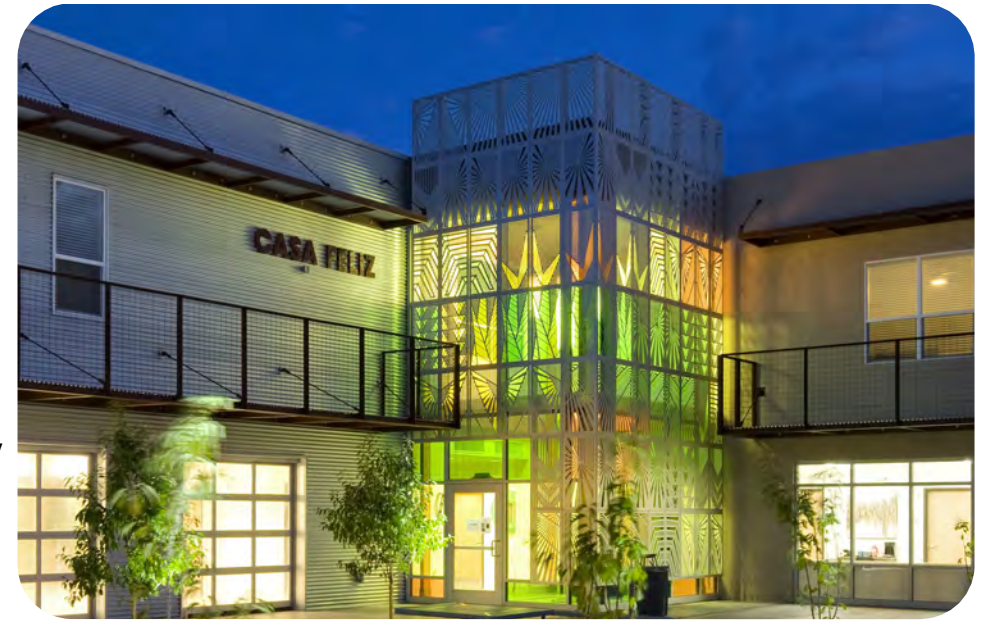
Casa Feliz's entry tower is wrapped in beautiful perforated aluminum panels depicting the many cultures represented in the International District
