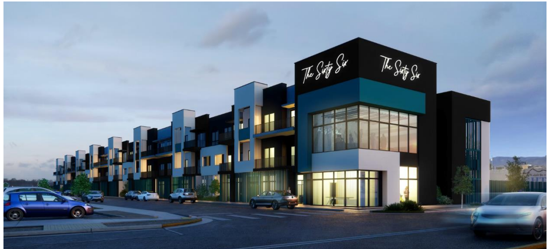
Façade facing Adams Street and Central Avenue
