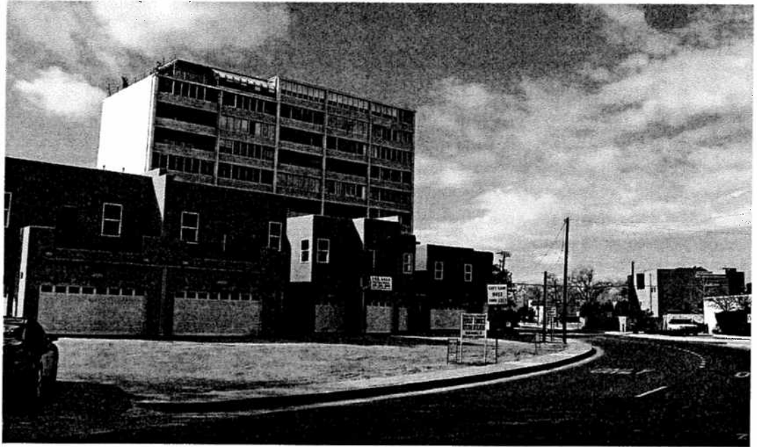
New project under construction to the northwest – R-3 Zoning
