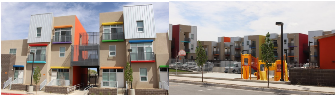
PLAZA CIUDANA- Located at 312 Indian School Rd NE, Albuquerque, NM 87102, the project consisted of the construction and management of a one, two, and three-story
