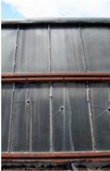
Wired skylight glazing.
