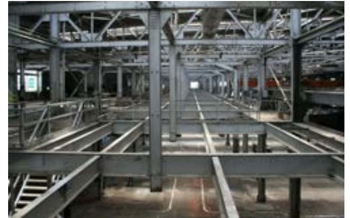
Longitudinal view from mezzanine catwalk.
