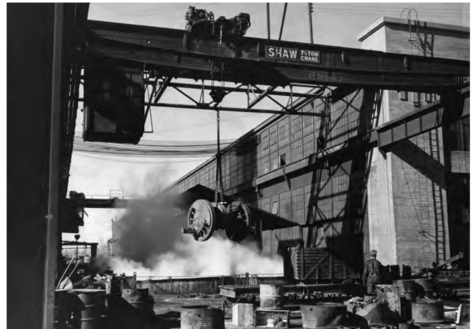
Bridge Crane in action circa~1943, Jack Delano Photographer, Farm Security Administration/Office of war information photograph collection (Library of Congress).
