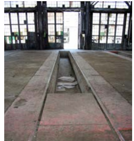
Erecting bay, floor trough.
