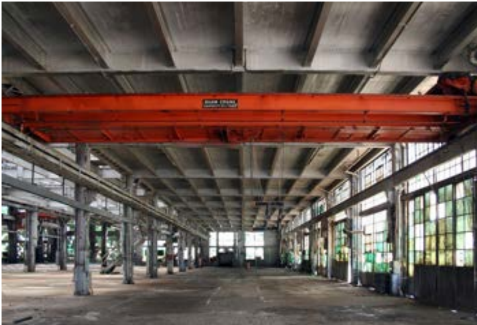
Machine Shop, bench bay - Below board formed, cast in place, concrete mezzanine.
