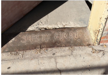
Safety signage, south washroom.
