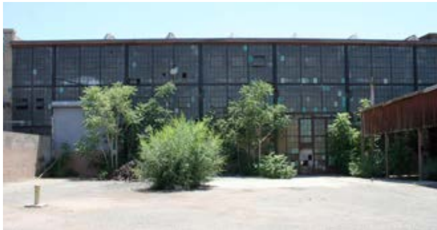
North elevation, exterior courtyard in foreground.
