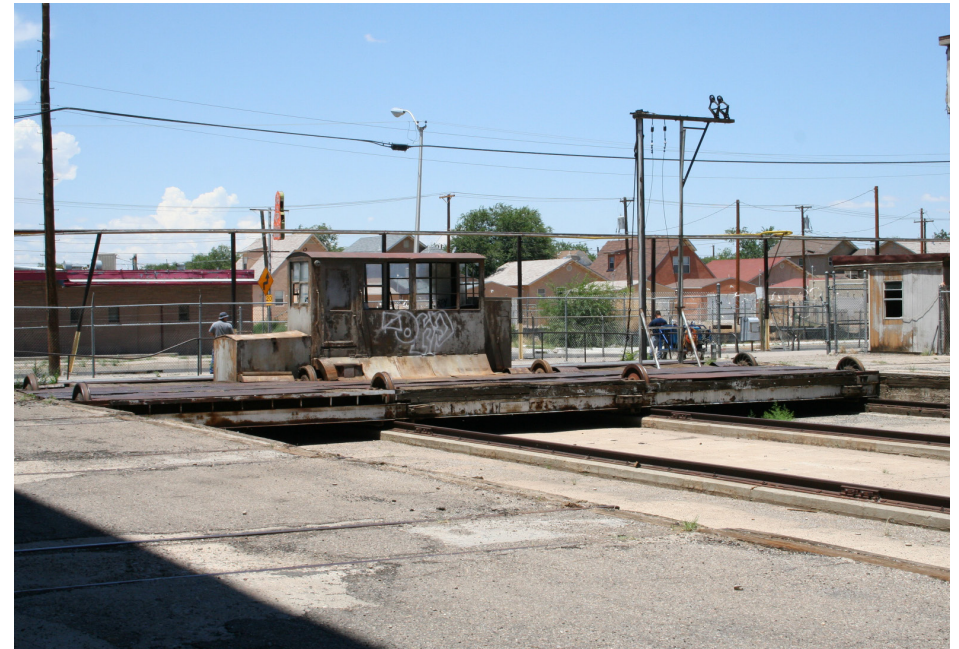
Transfer Table, west elevation.
