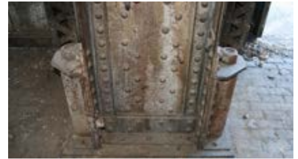
Erecting bay columns supported on deep piles, dampened by springs.
