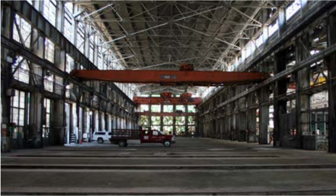
Machine Shop, erecting bay, 57' clear height to underside of truss structure. Floor troughs can be seen across slab.
