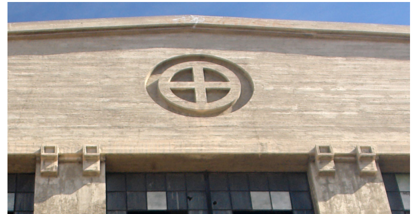
Cast-in-place concrete structure of Machine Shop with integral logo.
