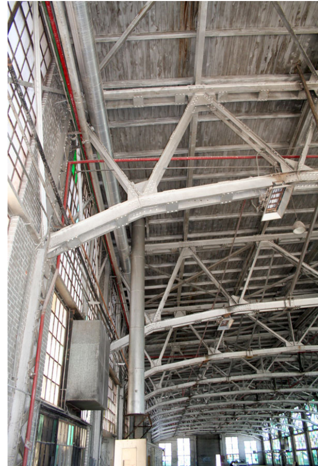
Blacksmith Shop, steel truss at column surrounded by masonry wall.
