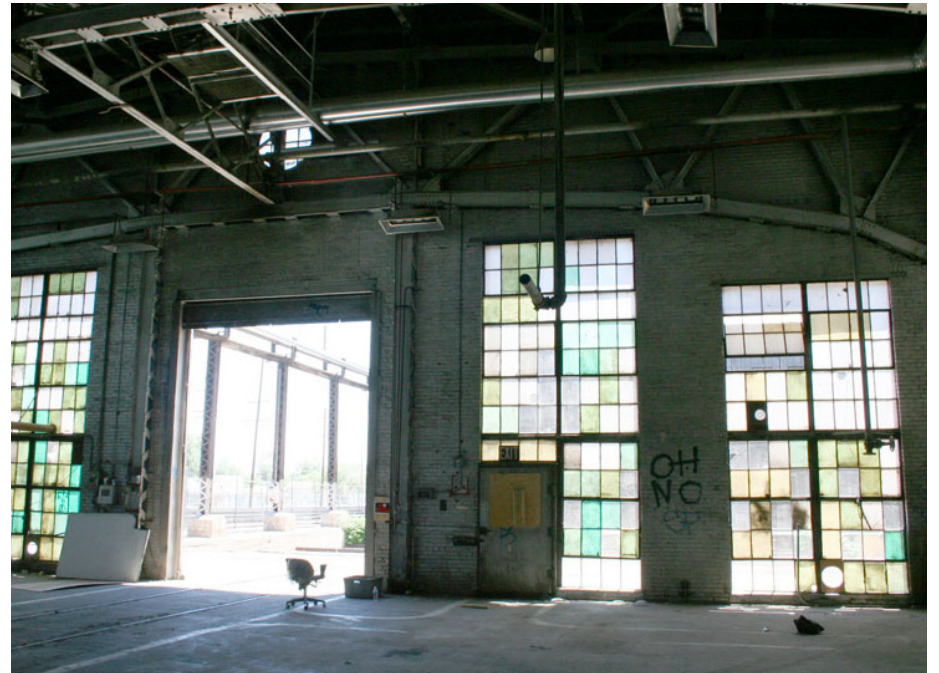
Interior view toward south elevation masonry wall.
