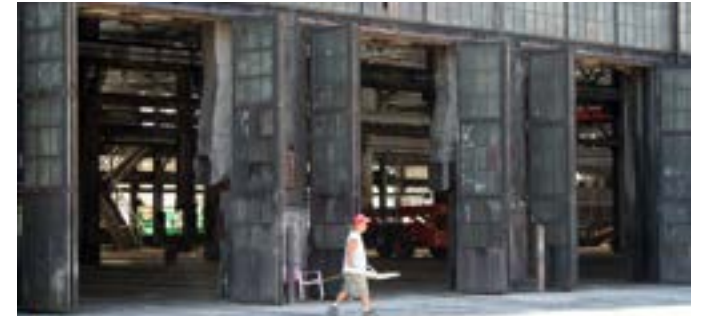
North elevation, operable doors.
