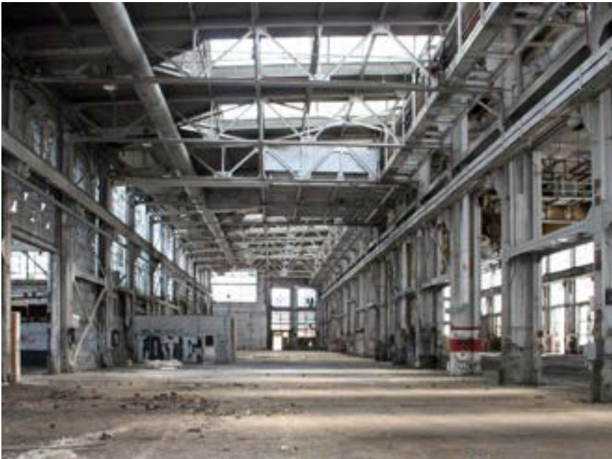
Boiler Shop, heavy equipment bay, pyramidal skylights
