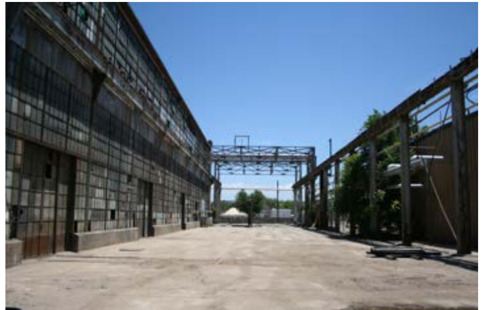
Bridge crane, view from west elevation.
