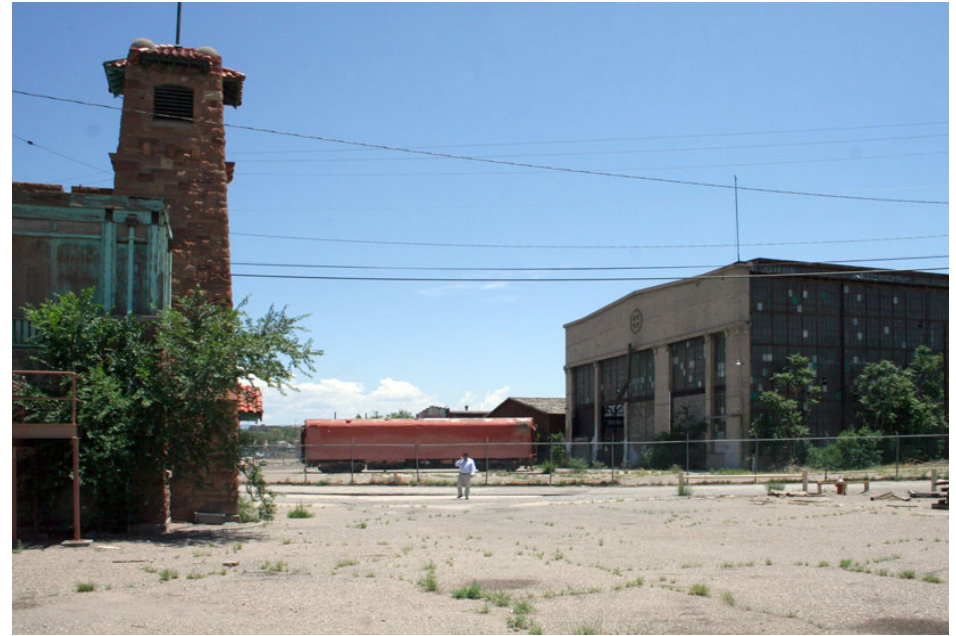
Southwest corner showing proximity to Tank Shop in background.
