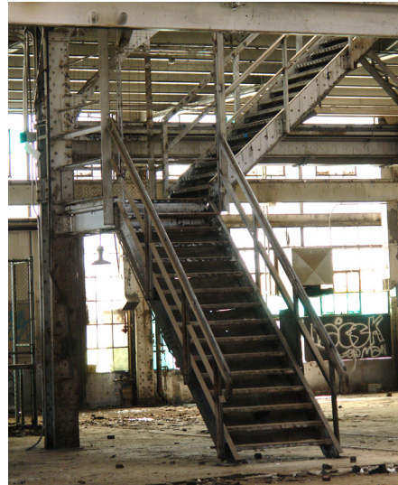
Machine Shop, stair to mezzanine.
