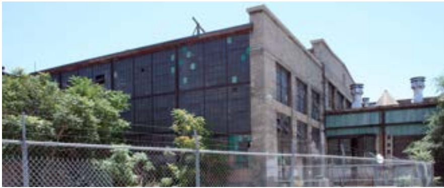
Northeast corner, reinforced concrete with fully glazed perimeter wall.
