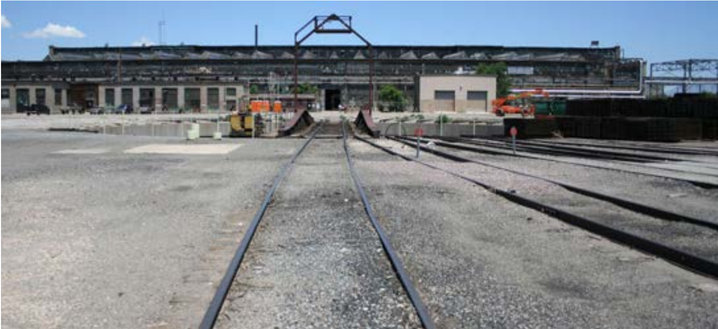
Machine Shop, south elevation, view across turntable.
