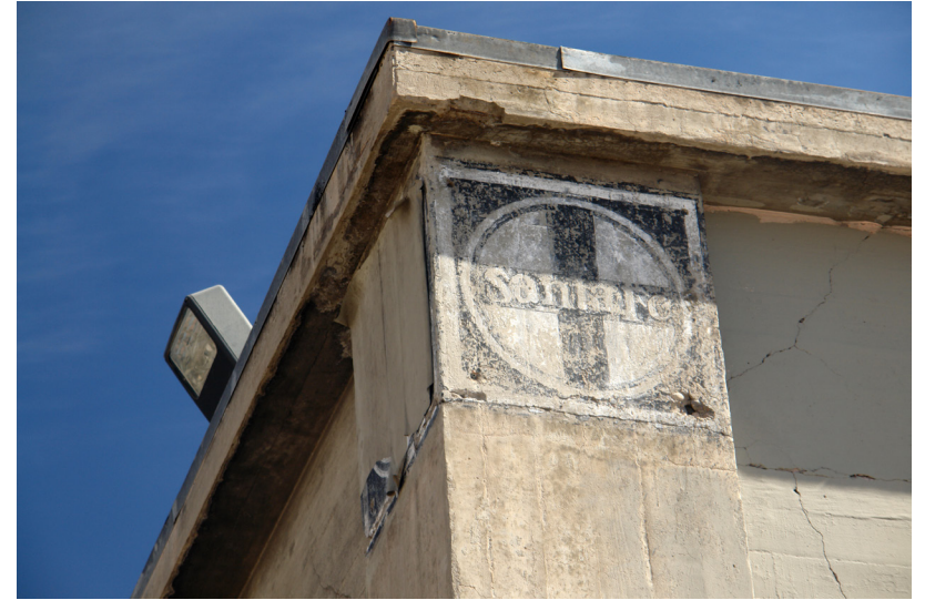
Cast-in-place concrete structure of Storehouse Building with painted logo.
