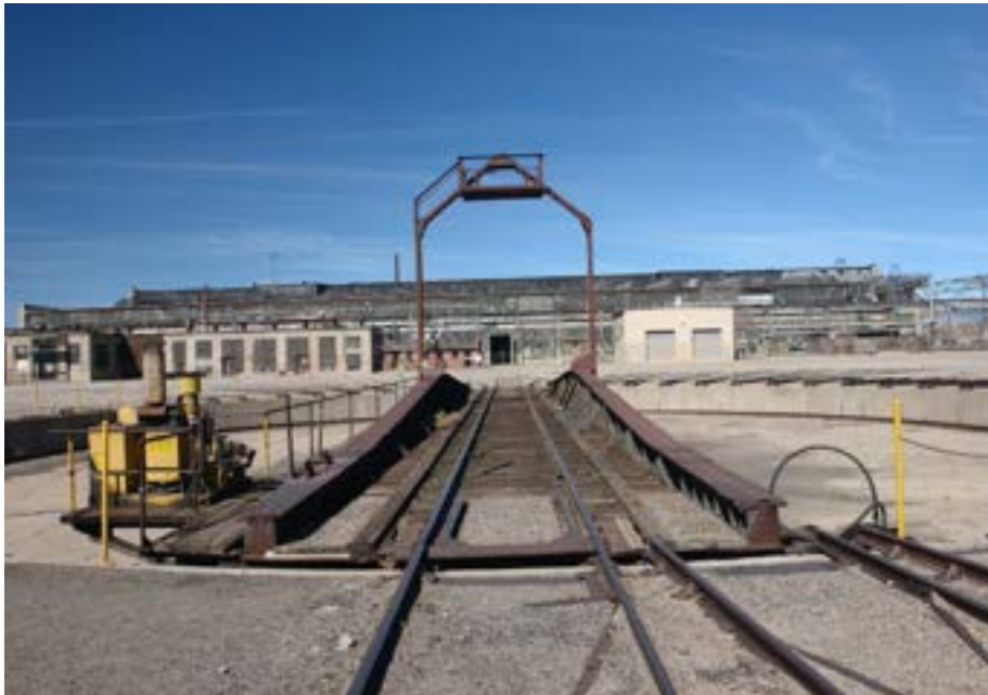
Turntable, view from south.
