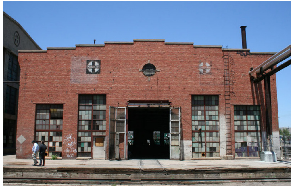
Blacksmith Shop, south elevation.
