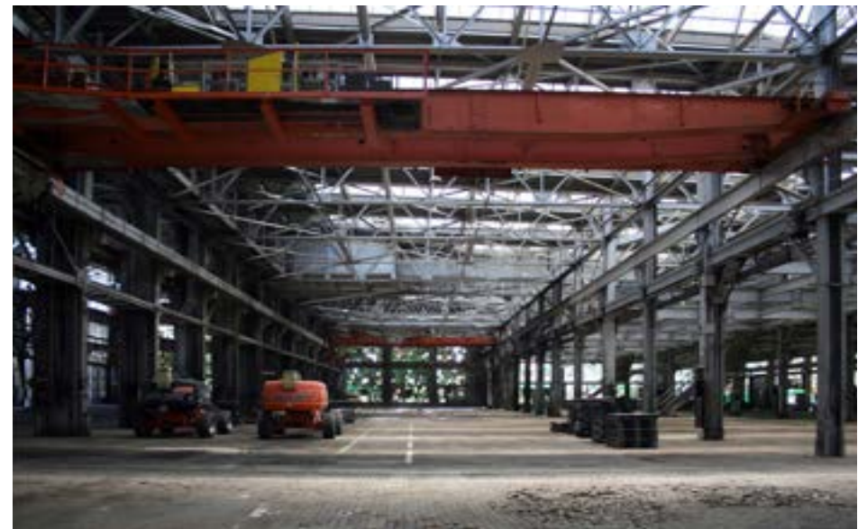
Machine Shop, heavy machinery bay.
