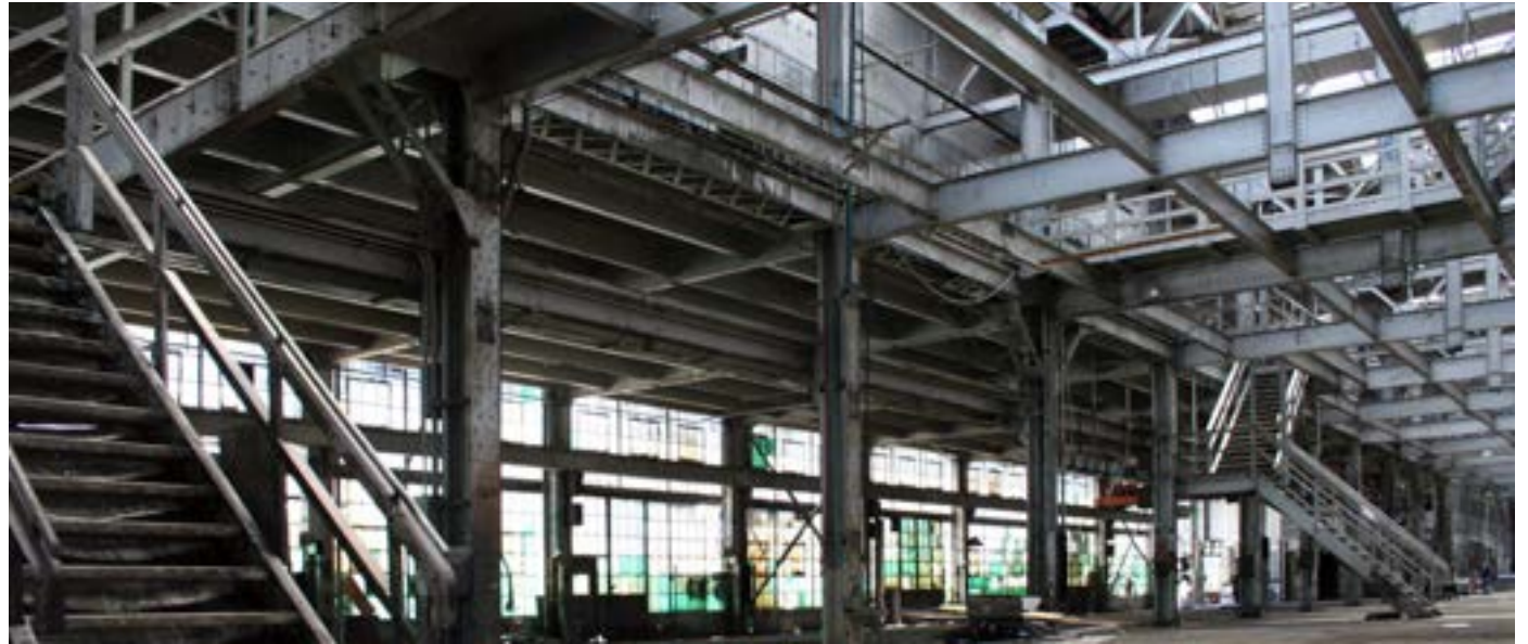
Machine Shop, view up toward mezzanine level.
