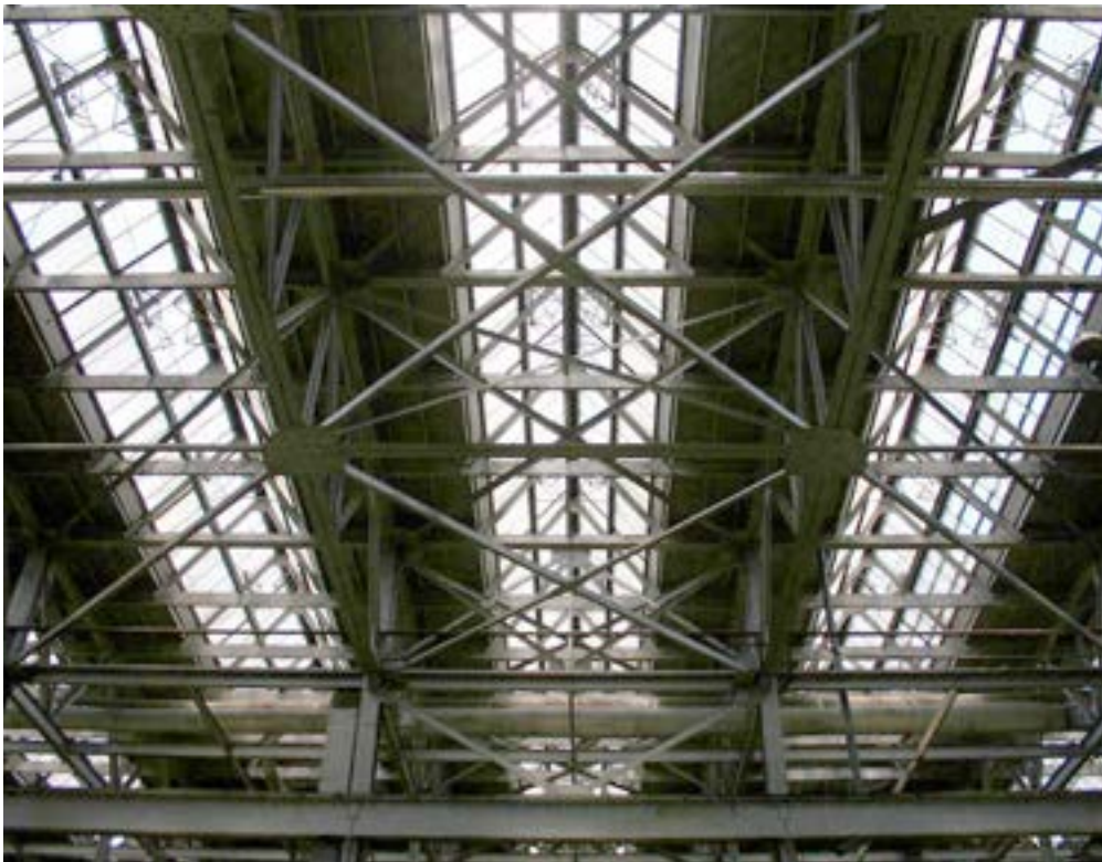
Machine Shop, pyramidal skylights over the heavy and light machinery bays.
