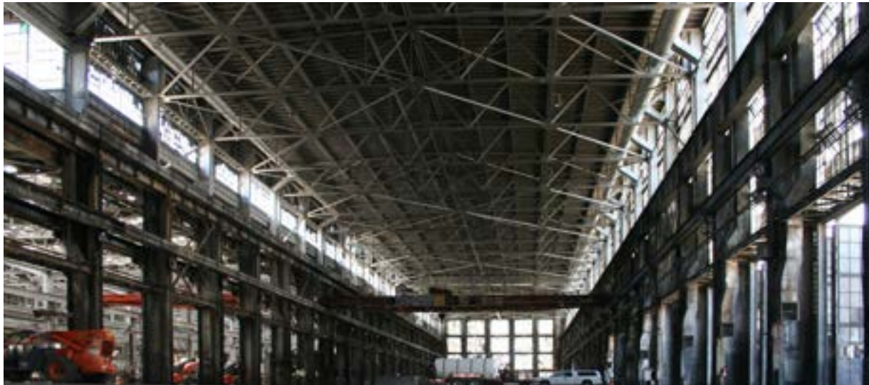
Machine Shop, erecting bay - view from within floor trough.
