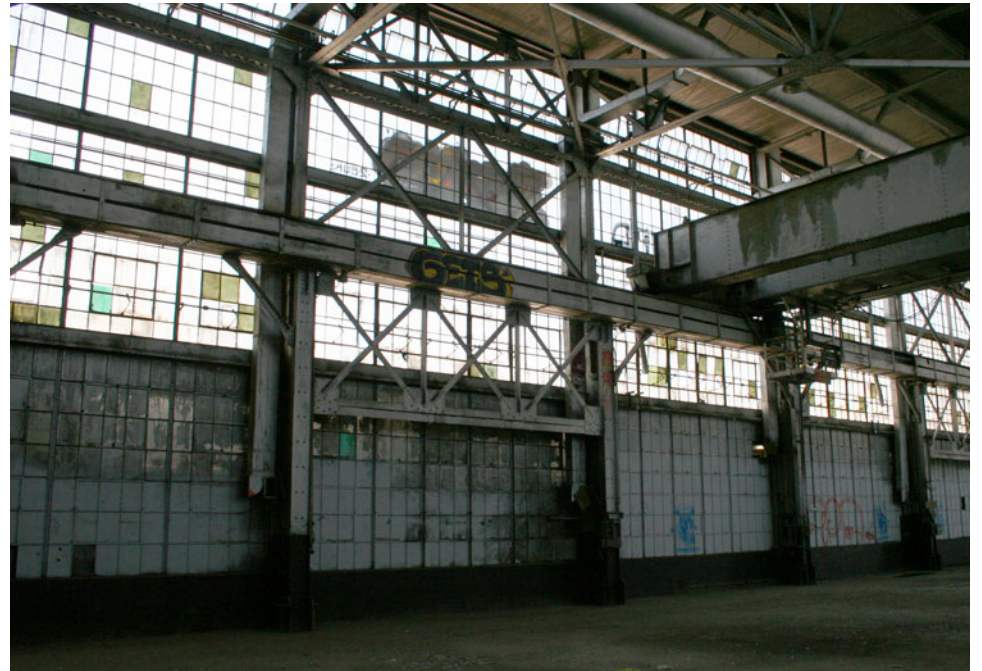
Interior view, west, fully glazed elevation.
