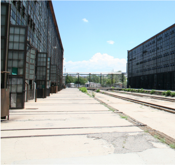
Rail lines adjacent to Transfer Table.
