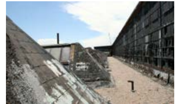
Clerestory skylight at erecting bay.
