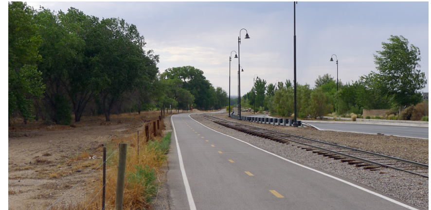
Circulation along the Bosque includes a narrow gauge rail line and pedestrian/bike path.
