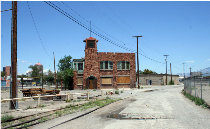
Firehouse, south elevation.
