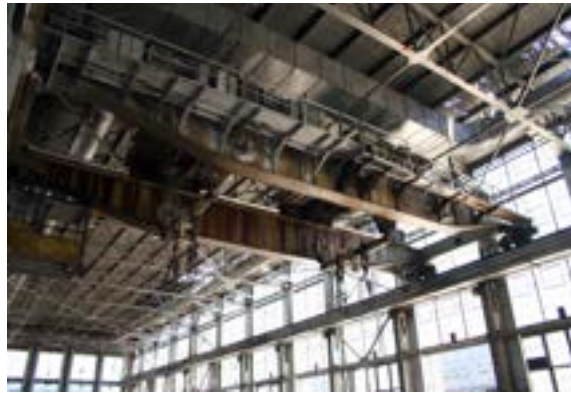
Boiler Shop, cranes in erecting bay.
