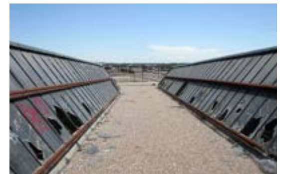
Built-up roofing, positive slope to south.
