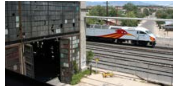
Southeast corner, adjacent to active BNSF rail lines.
