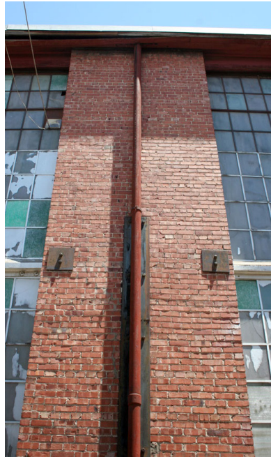
West/east elevation, steel plate upgrades.
