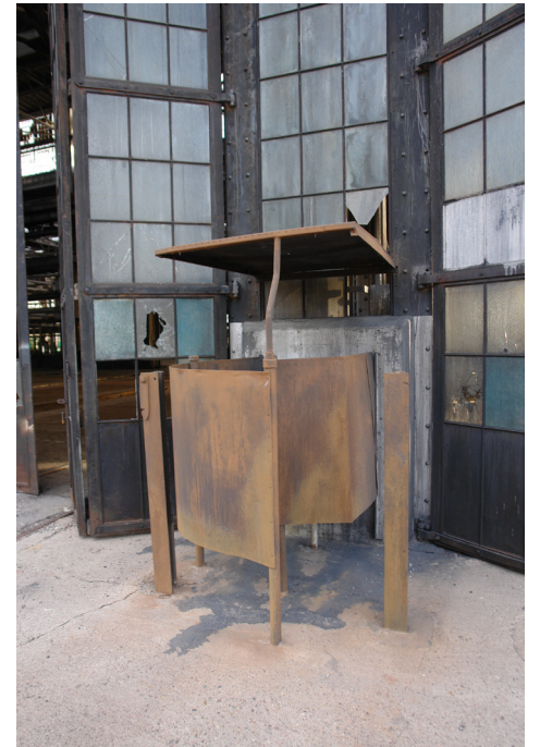
Machine Shop, urinals.
