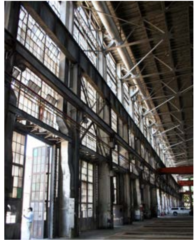
North interior elevation showing large operable doors.
