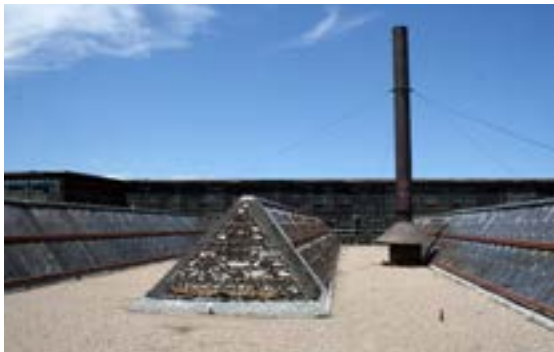
Machine Shop, view from roof looking north.
