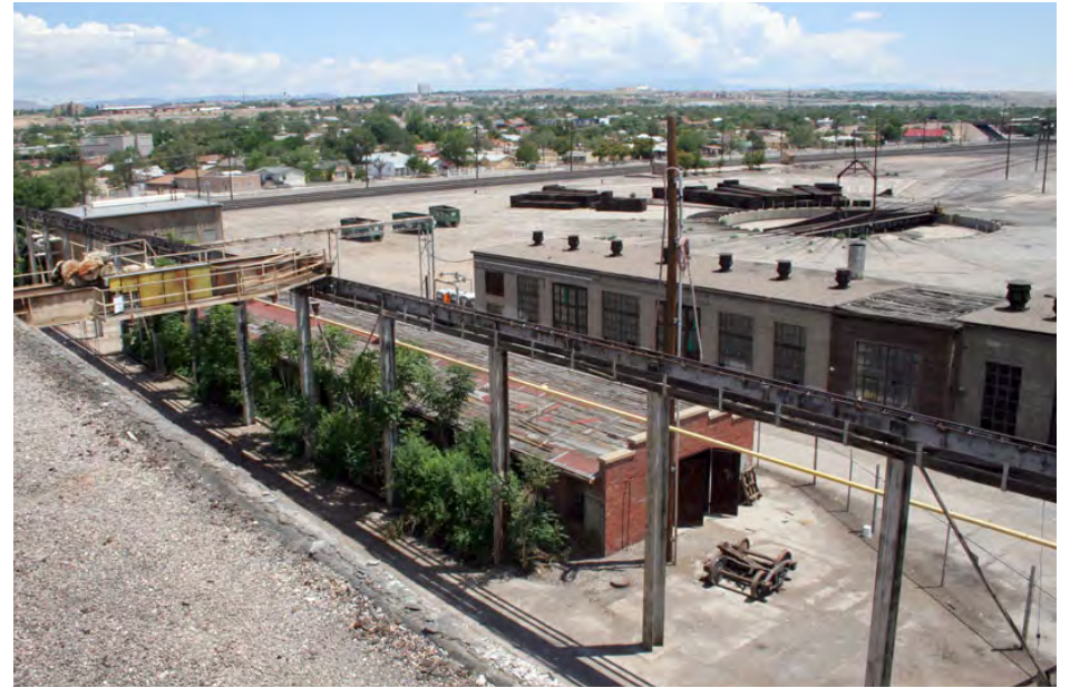
View east toward South Broadway neighborhood from roof of Machine Shop.
