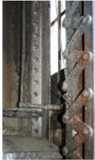
Crank mechanism for skylight operation.
