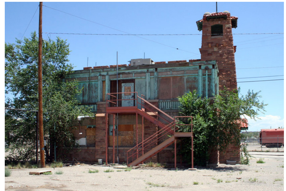
Firehouse, west elevation.
