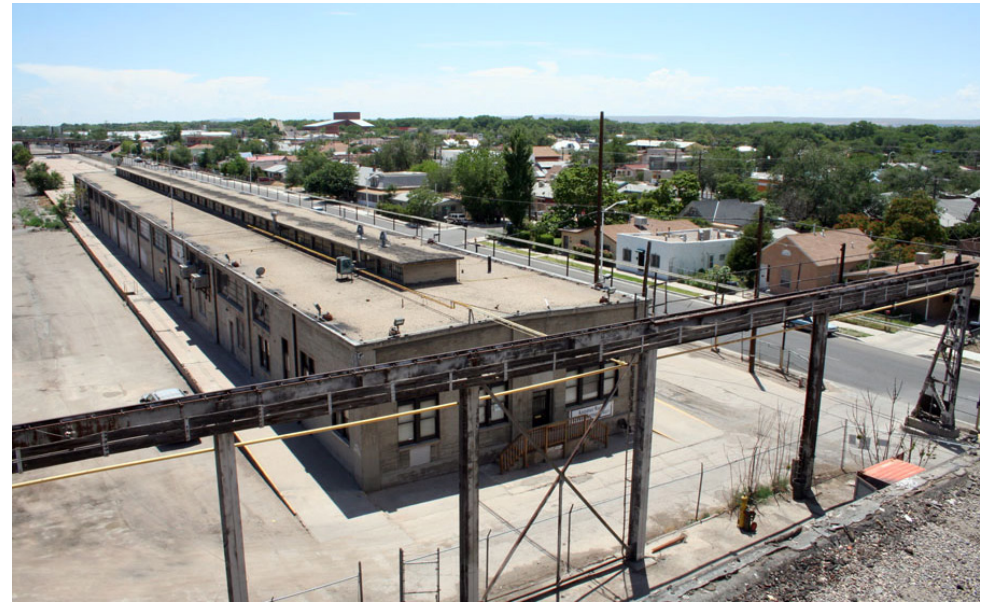
Aerial view of the Storehouse from roof of the Machine Shop.
