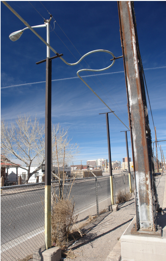
Perimeter street lighting and welding lines.
