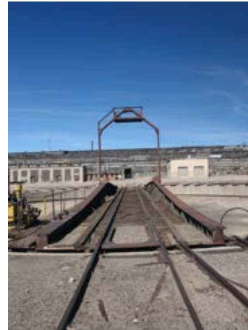
Turntable, view from south.
