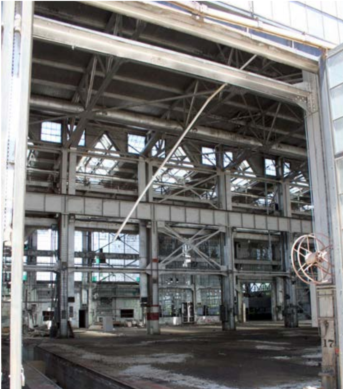
Boiler Shop, view from south operable doors.
