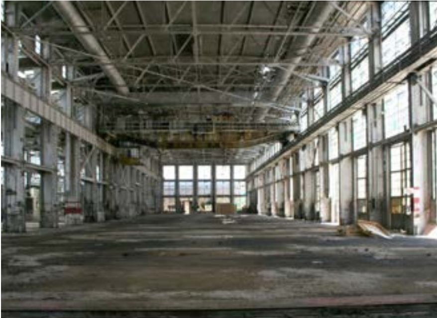
Boiler Shop, erecting bay, fully glazed southern elevation, crane at rear. Floor troughs seen across floor.
