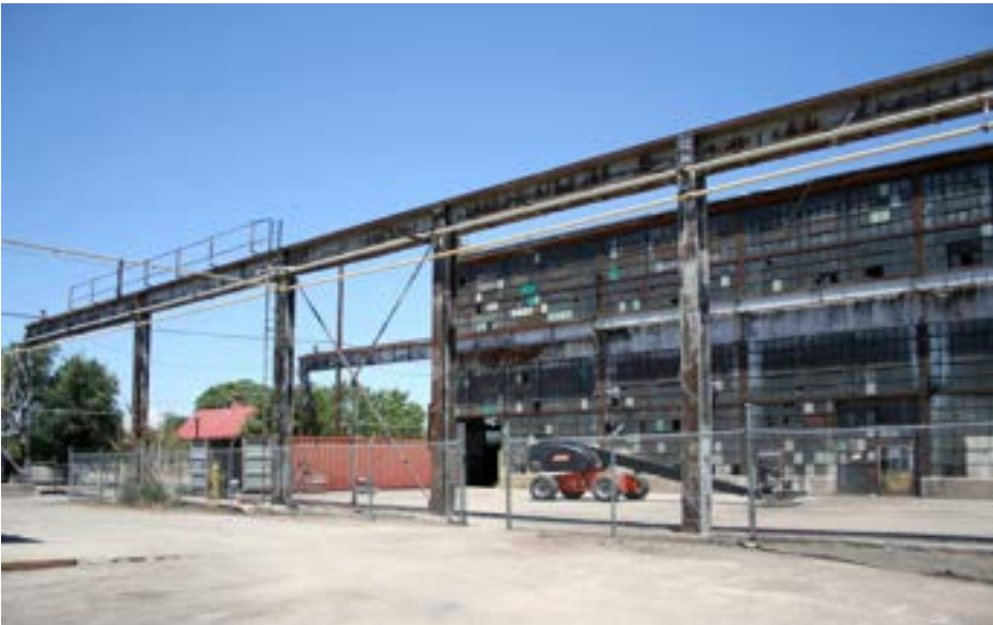
South bay, crane runway, exterior loading crane.
