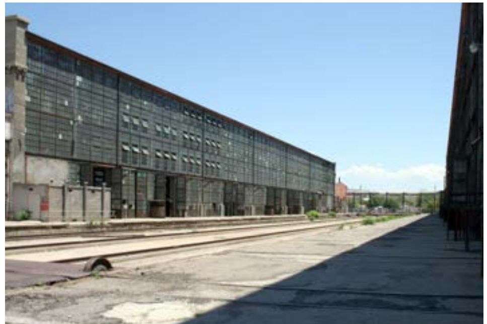
Boiler Shop, south elevation, view from Transfer Table.
