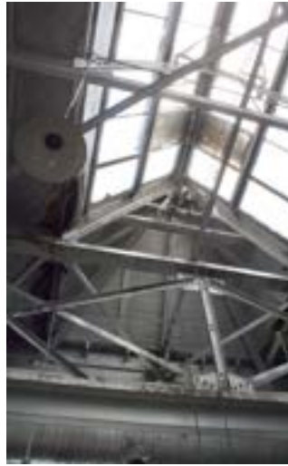
Gear/pulley mechanism for skylight operation.
