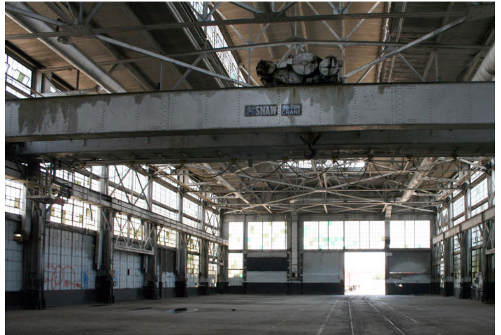
Tank Shop, interior view, central bay with Shaw 30-ton crane in foreground.
