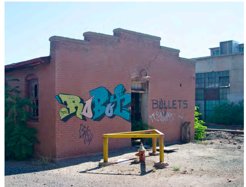
Current condition (2014) of Rail Yards buildings.
