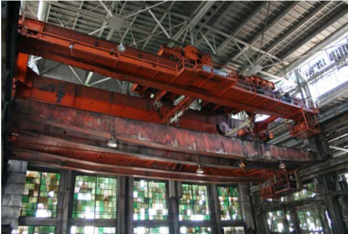
Machine Shop, erecting bay, main 250 ton crane.
