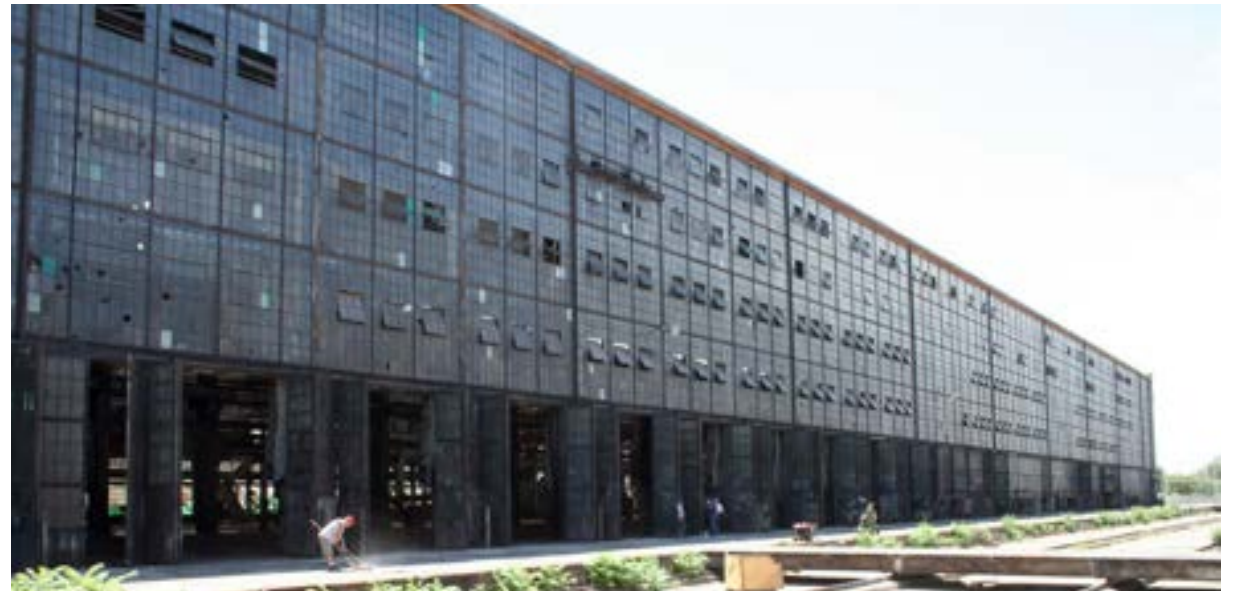
Machine Shop, north elevation, view from Transfer Table.
