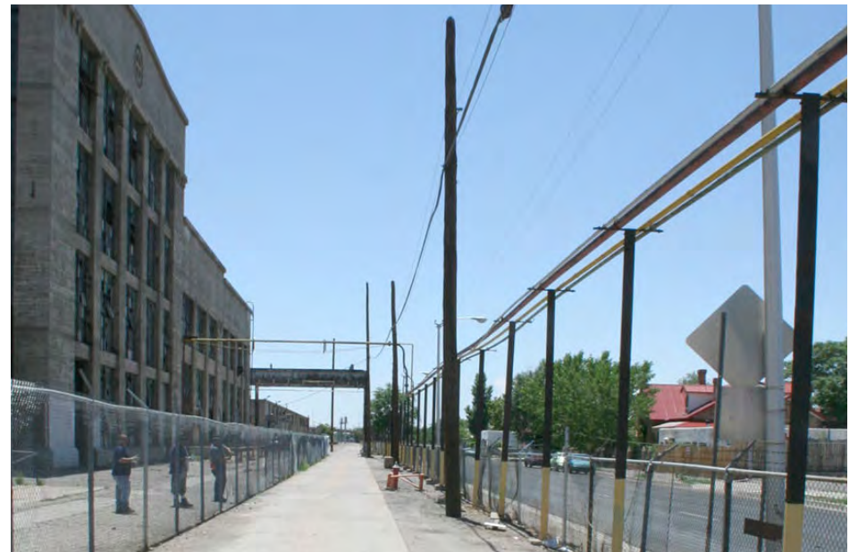
View south down fire runway between Machine Shop and Barelas neighborhood to the west.
