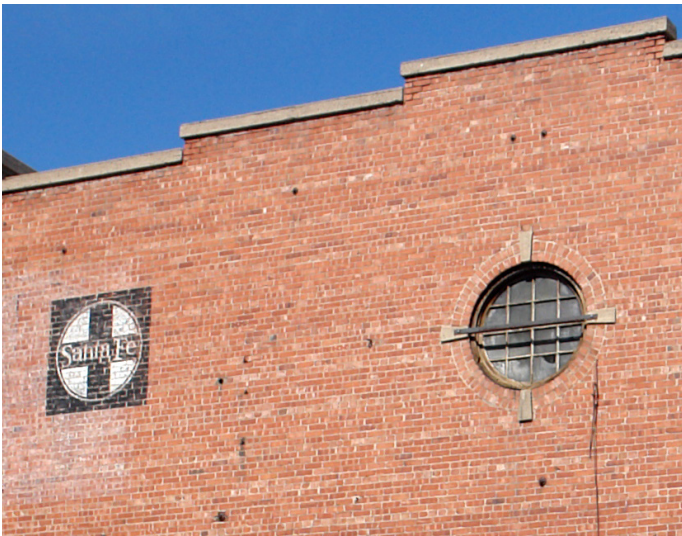
Masonry facade of Blacksmith Shop with painted and integral logo/window.
