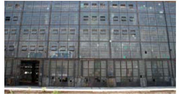
North elevation, completely glazed façade.
