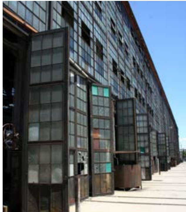
North elevation, operable doors.
