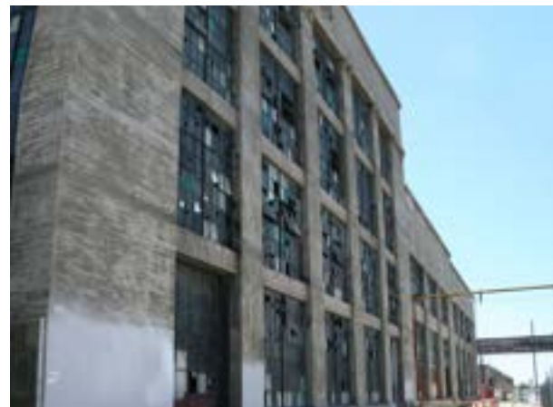
West elevation, cast in place concrete frame.
