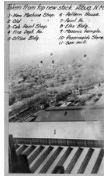
View from atop Smokestack.
