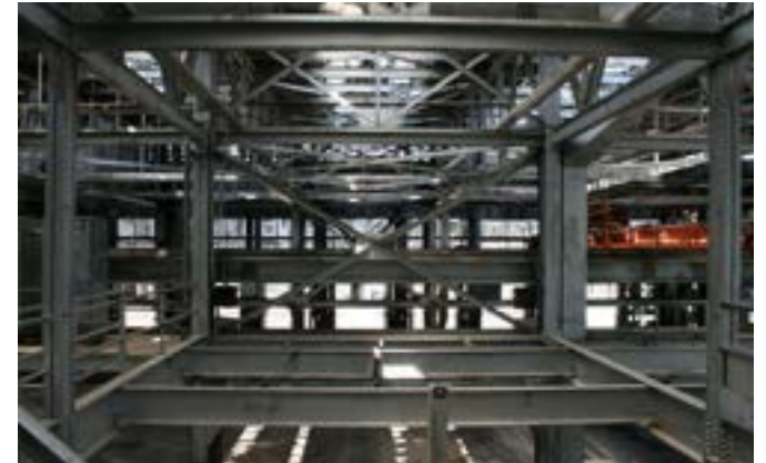
Transverse view from mezzanine.
