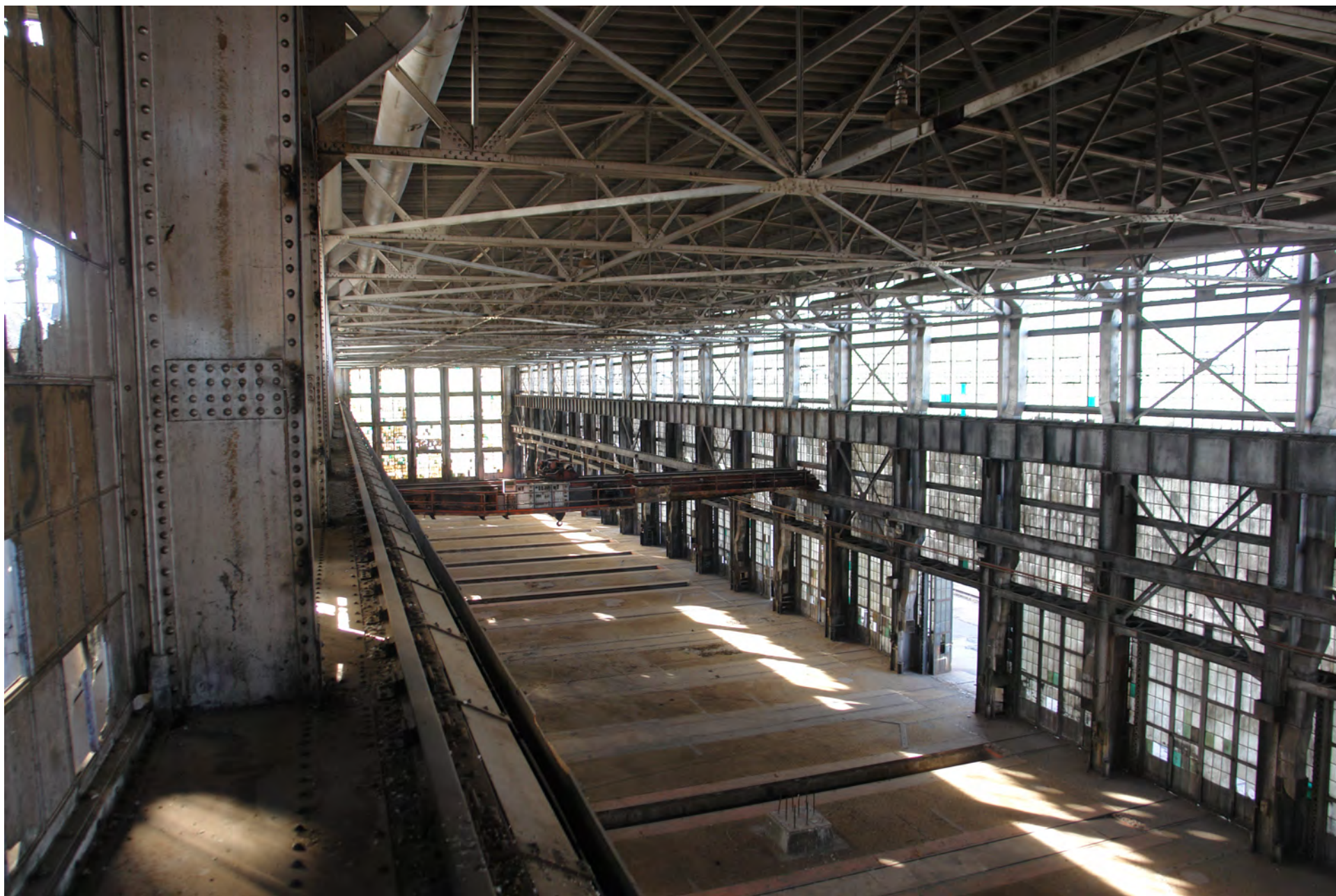
Figure 3: Spirit of Place Machine Shop interior.
