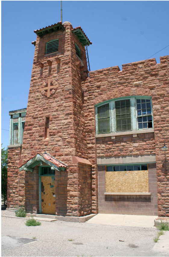
Firehouse, south elevation - detail.
