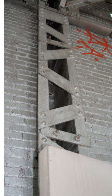
Steel 'trussed' column.
