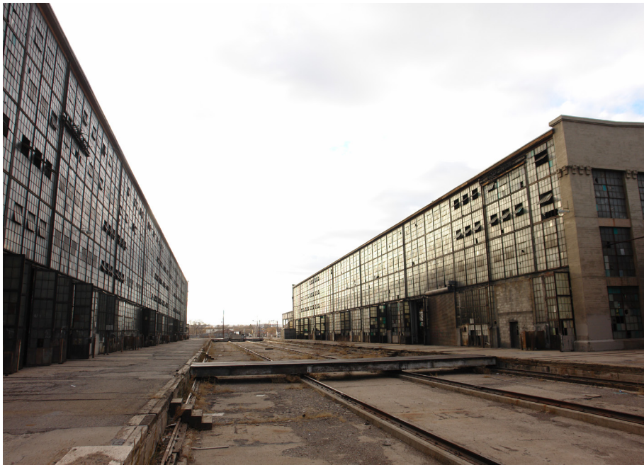
Transfer Table, view from east side.
