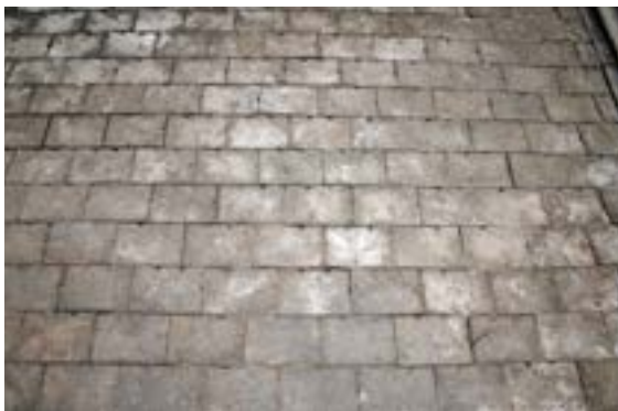
Flooring, 3" thick creosoted end-grain wood blocks.
