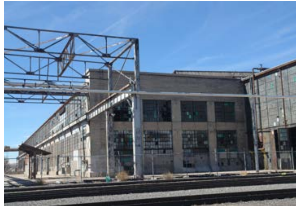
Bridge crane, view from east elevation.
