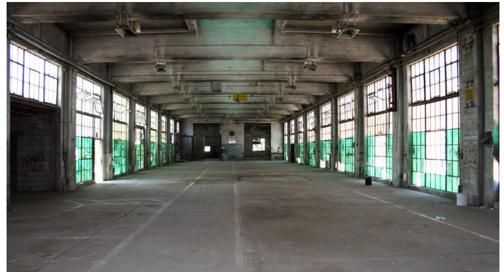
Flue Shop, view down center of bay.
