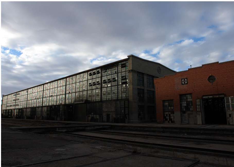
Transfer Table, view from the southeast corner to Blacksmith Shop and Boiler Shop.
