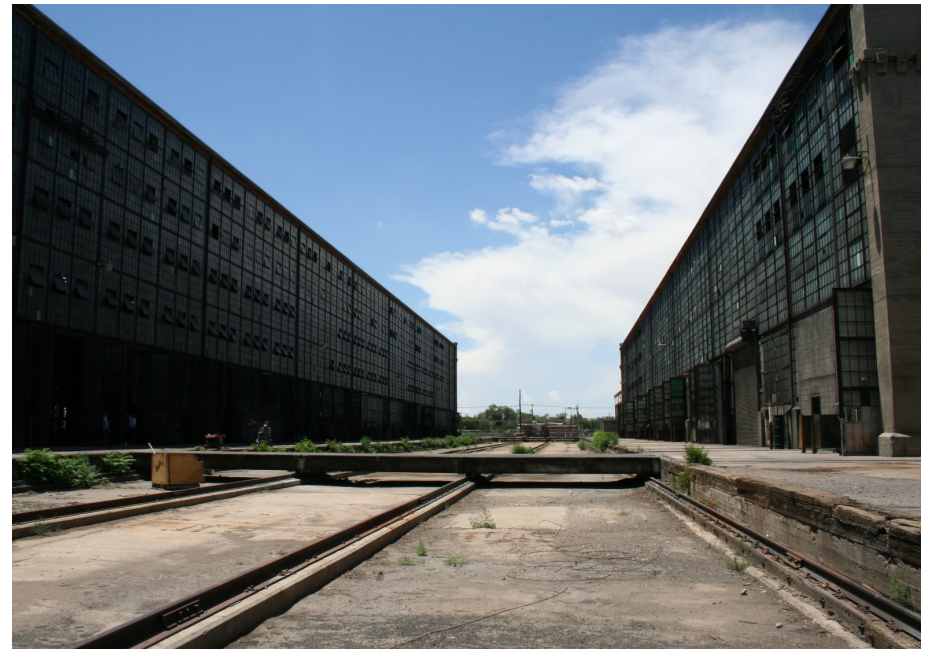
Transfer Table, view from the east side.
