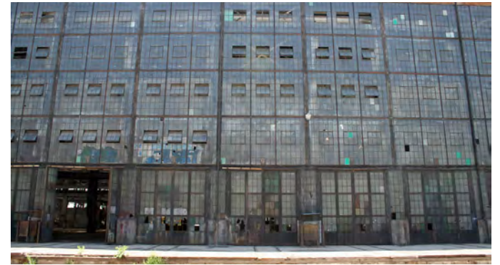
North elevation, completely glazed façade.
