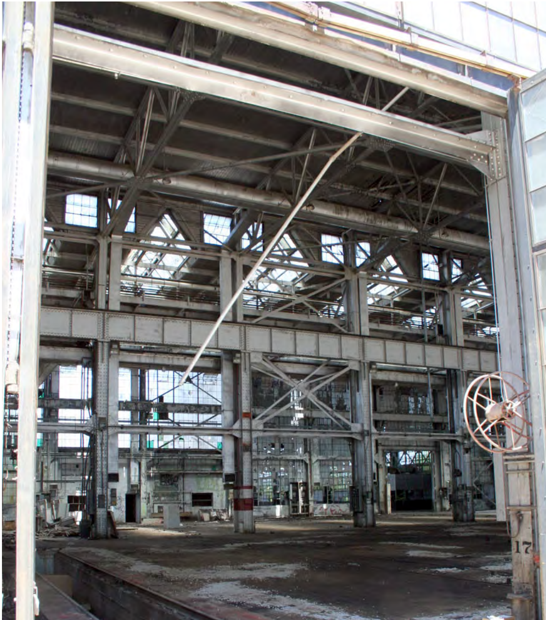
Boiler Shop, view from south operable doors.
