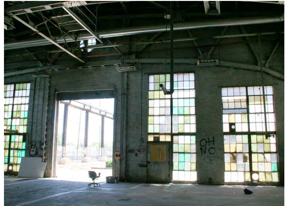
Interior view toward south elevation masonry wall.
