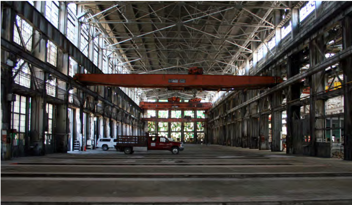
Machine Shop, erecting bay, 57' clear height to underside of truss structure. Floor troughs can be seen across slab.
