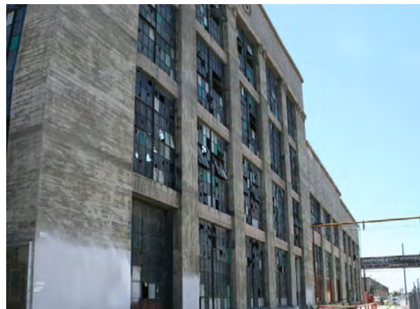
West elevation, cast in place concrete frame.
