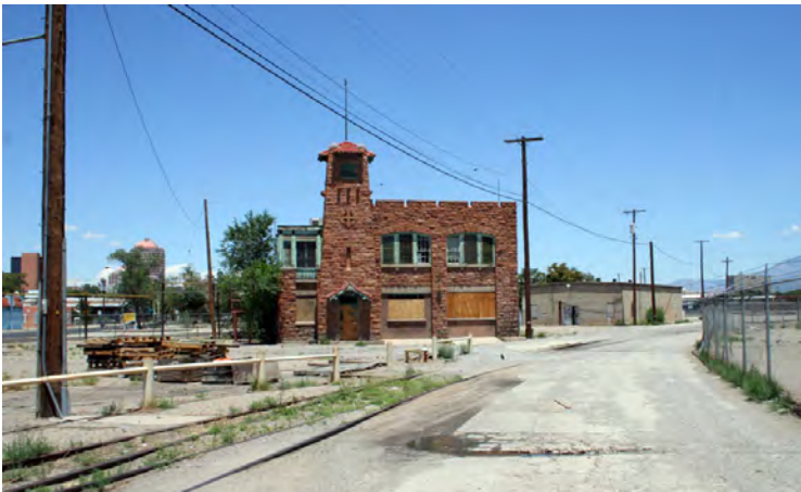
Firehouse, south elevation.
