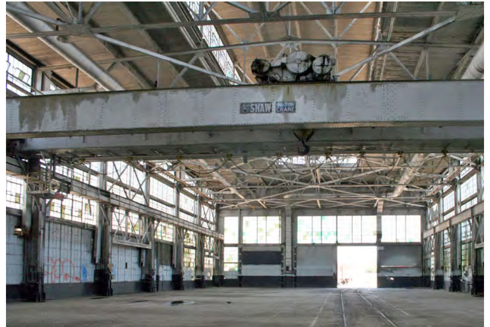
Tank Shop, interior view, central bay with Shaw 30-ton crane in foreground.
