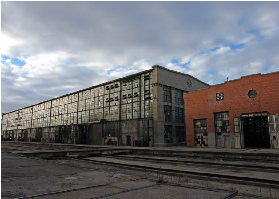
Transfer Table, view from the southeast corner to Blacksmith Shop and Boiler Shop.
