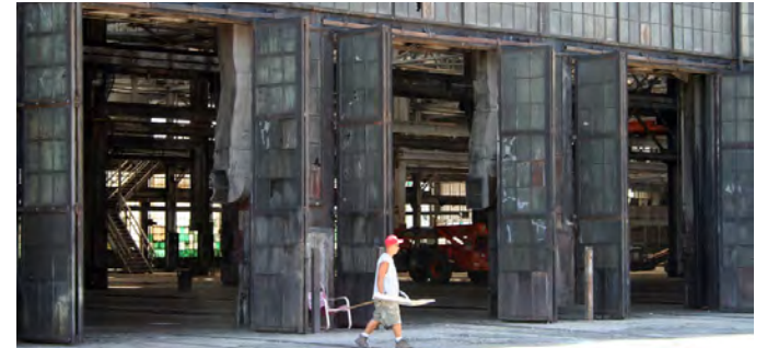
North elevation, operable doors.
