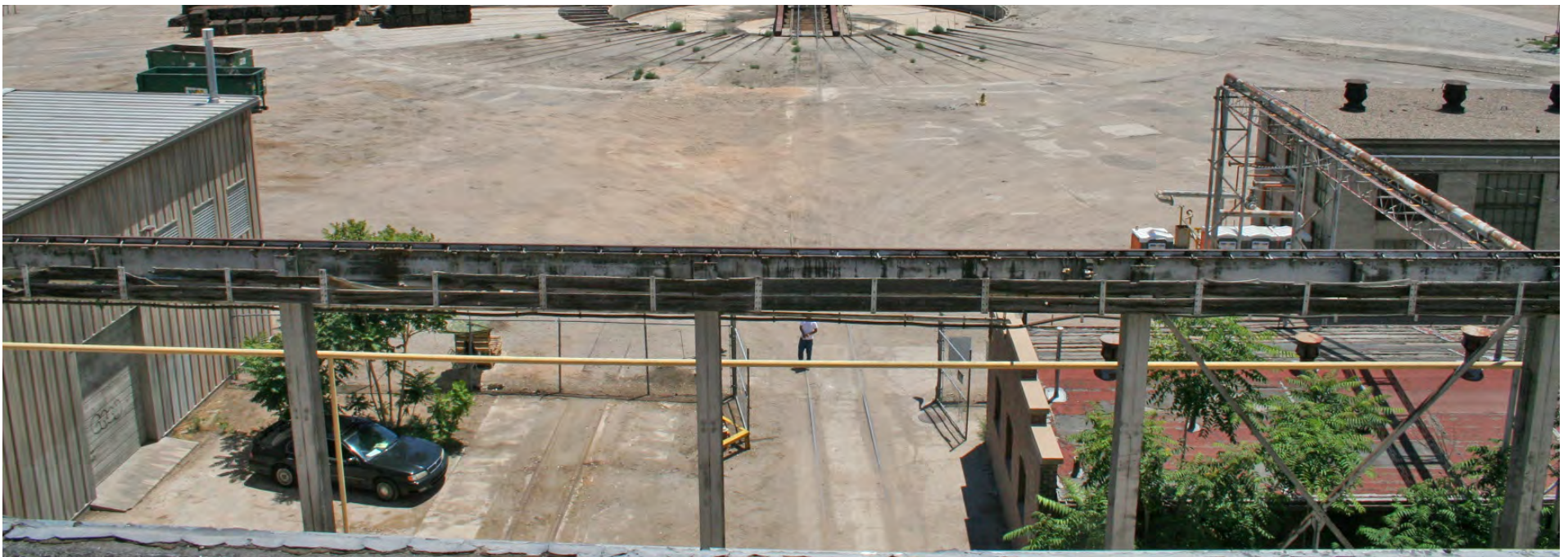
Bridge crane, view from Machine Shop roof, north towards south.
