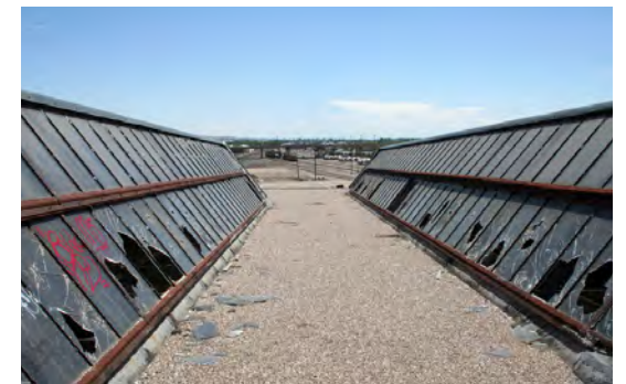
Built-up roofing, positive slope to south.
