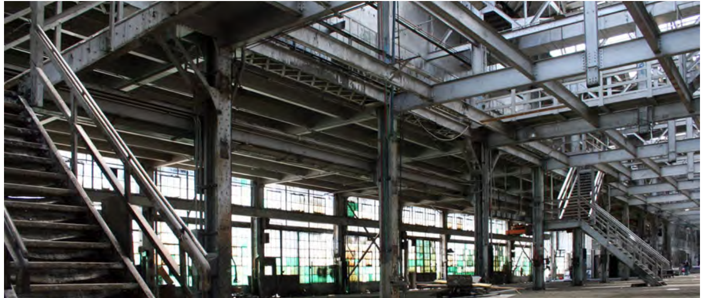
Machine Shop, view up toward mezzanine level.
