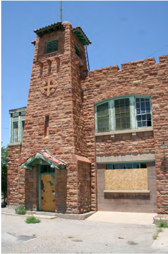
Firehouse, south elevation - detail.
