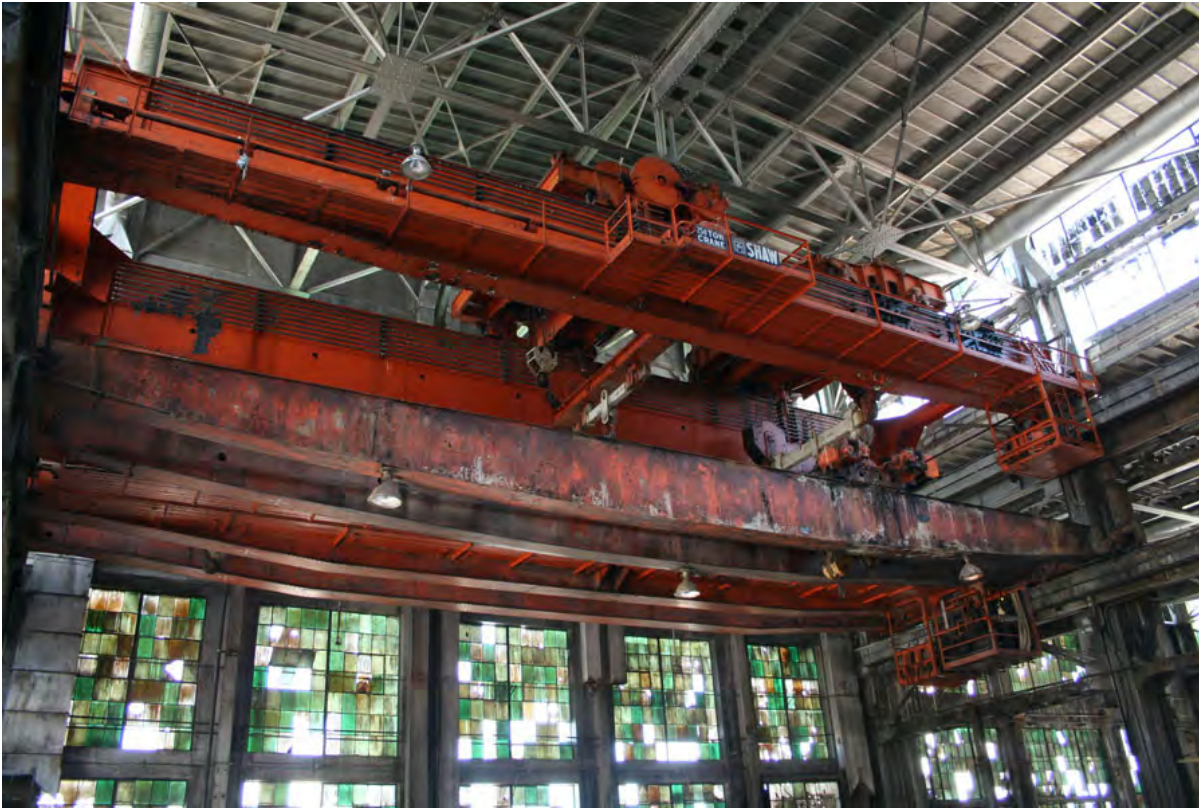
Machine Shop, erecting bay, main 250 ton crane.
