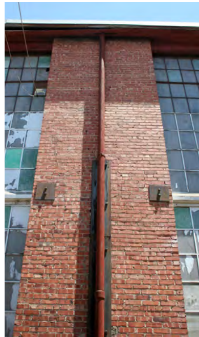
West/east elevation, steel plate upgrades.
