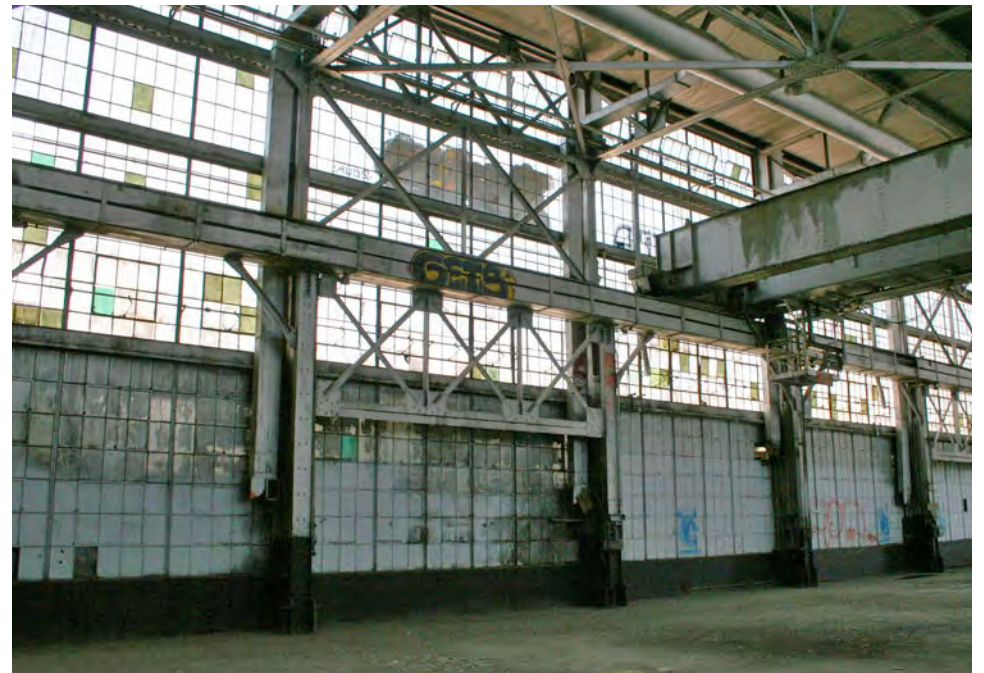
Interior view, west, fully glazed elevation.
