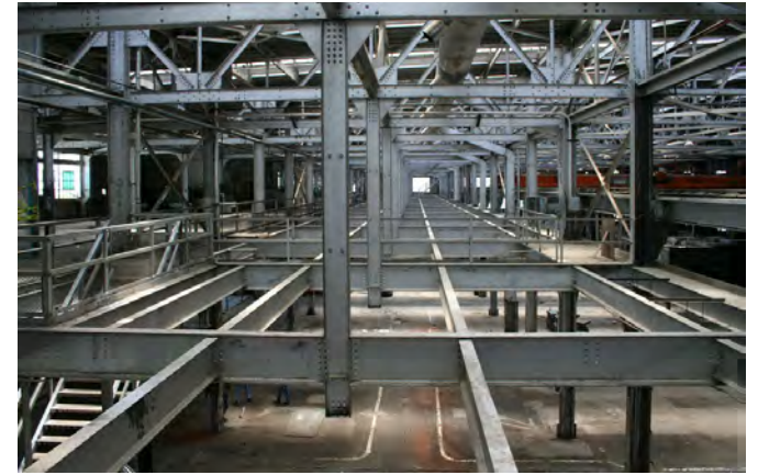
Longitudinal view from mezzanine catwalk.
