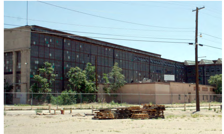
Northwest corner, Cab Paint Shop in the foreground.
