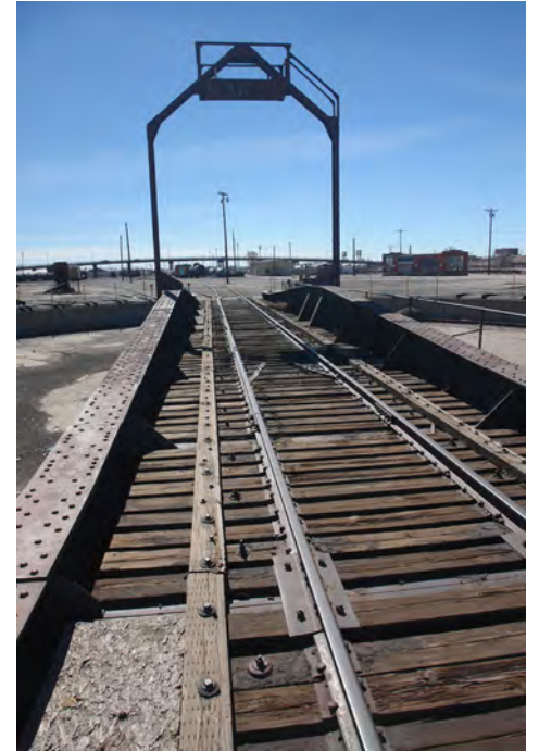
Turntable, steel rail tracks and wood railroad ties.
