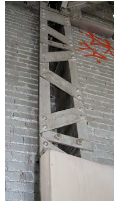
Steel 'trussed' column.
