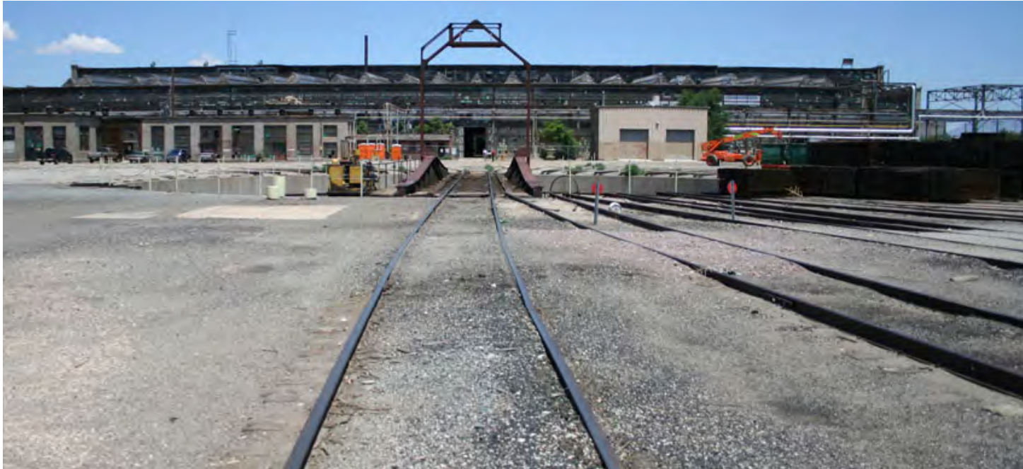
Machine Shop, south elevation, view across turntable.
