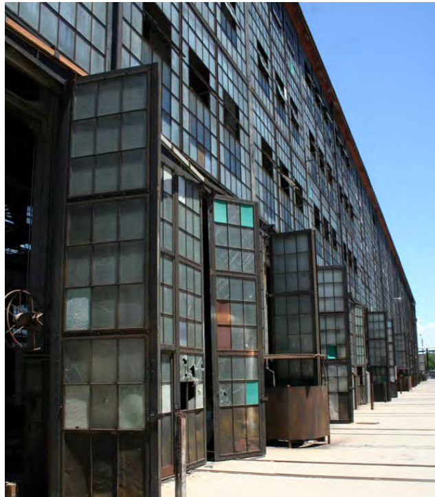
North elevation, operable doors.
