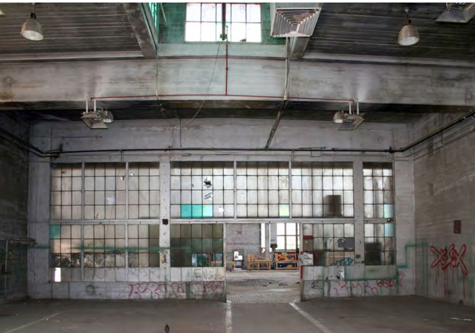
Flue Shop, Interior view of entrance, Boiler shop shown beyond.
