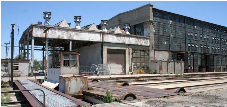
Firing shed attached to west elevation, Transfer Table in foreground.
