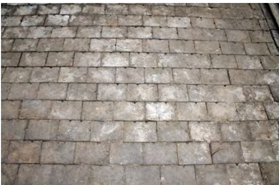
Flooring, 3" thick creosoted end-grain wood blocks.
