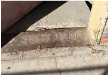
Safety signage, south washroom.
