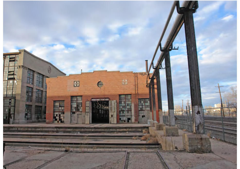
Transfer Table, view from southeast corner to Blacksmith Shop and Boiler Shop.
