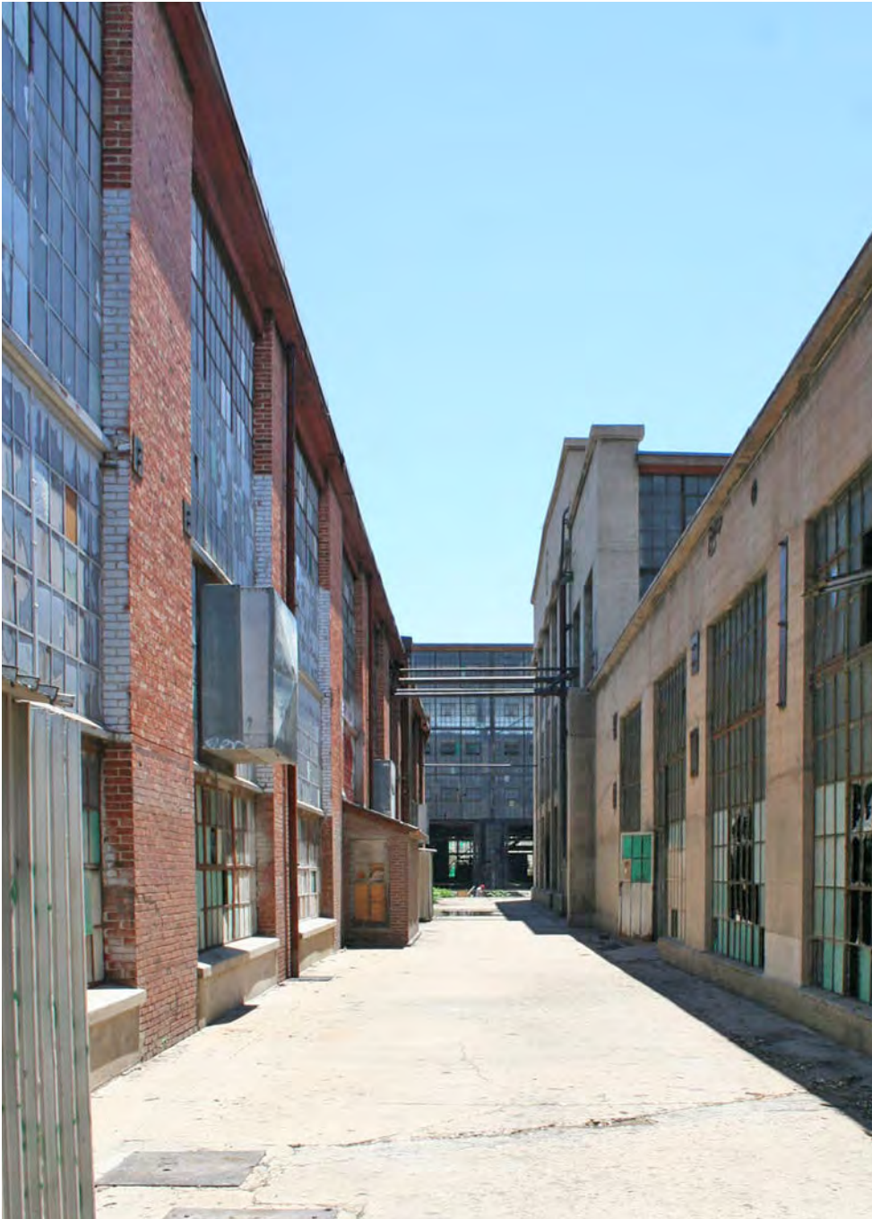
Exterior walkway between Blacksmith Shop (Left) and Flue Shop (Right), Machine Shop/Transfer Table shown in background.
