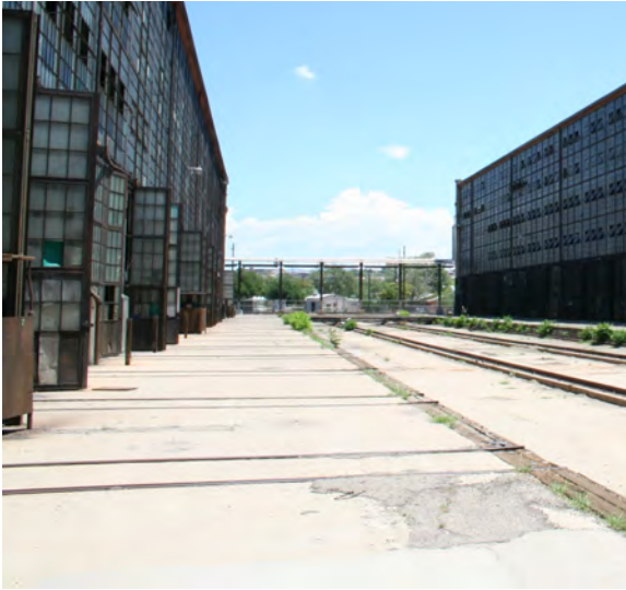
Rail lines adjacent to Transfer Table.
