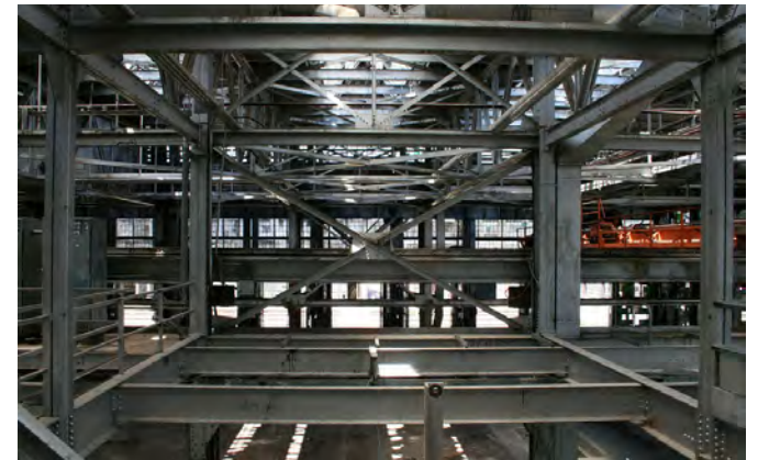
Transverse view from mezzanine.
