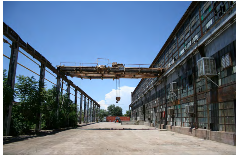
15 ton bridge crane connected to south elevation of Machine Shop.
