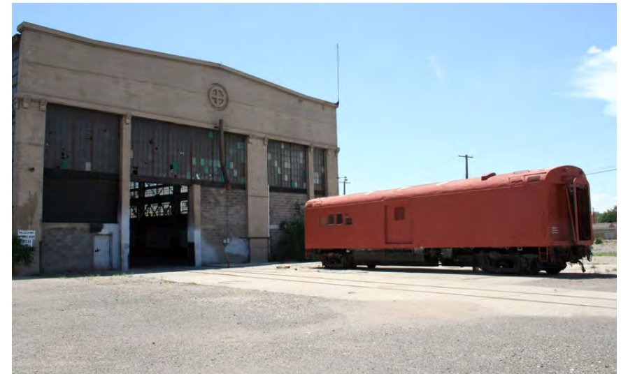
Tank Shop, north elevation.
