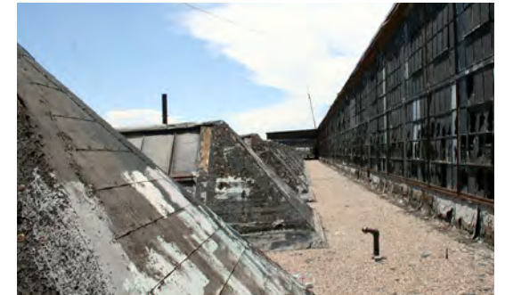
Clerestory skylight at erecting bay.
