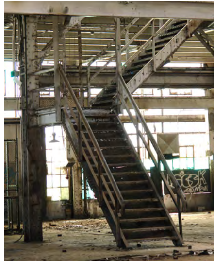
Machine Shop, stair to mezzanine.
