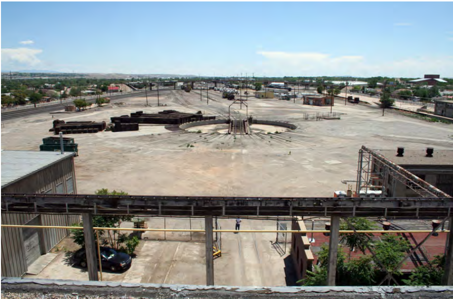
View south toward former site of Roundhouse building from roof of Machine Shop. Turntable is still in operation.
