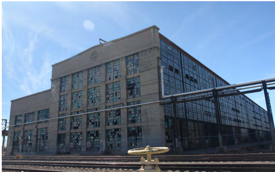
Machine Shop, view towards east elevation.
