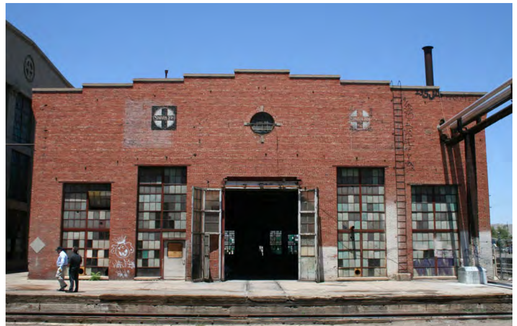
Blacksmith Shop, south elevation.
