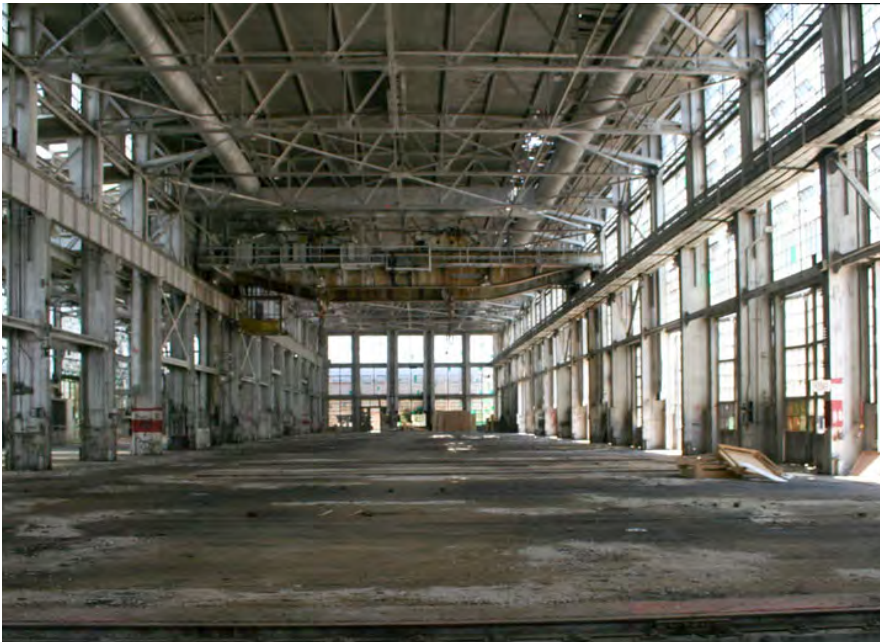
Boiler Shop, erecting bay, fully glazed southern elevation, crane at rear. Floor troughs seen across floor.
