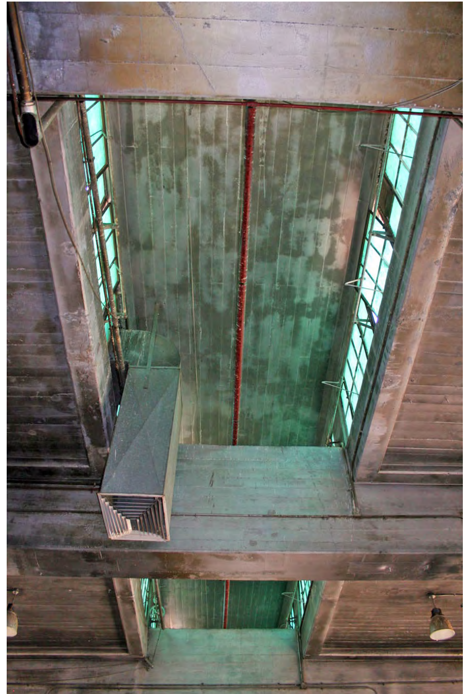
Flue Shop, View up toward operable clerestory windows.
