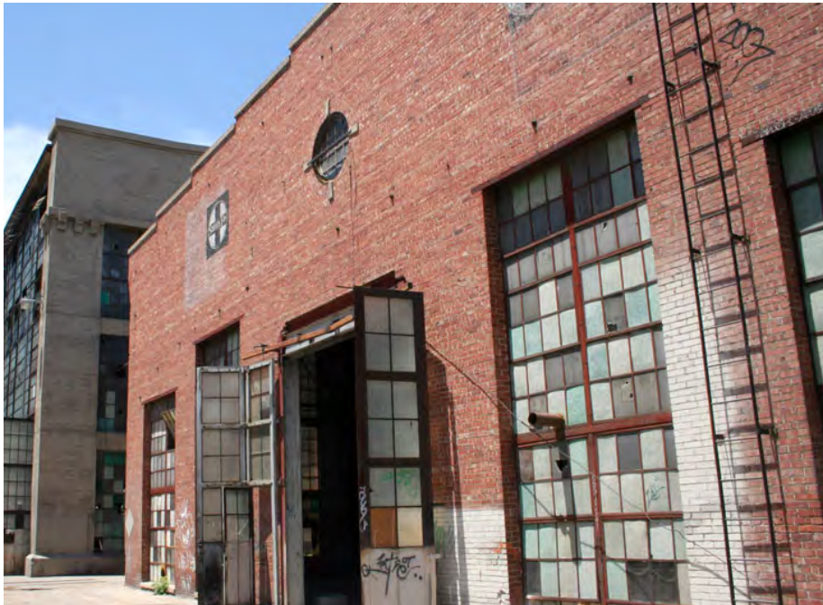
South elevation showing proximity to Boiler Shop to the west.
