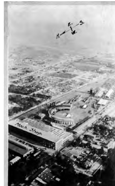
Rail Yards upon completion of Machine Shop, ~1922
