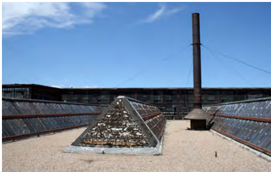
Machine Shop, view from roof looking north.
