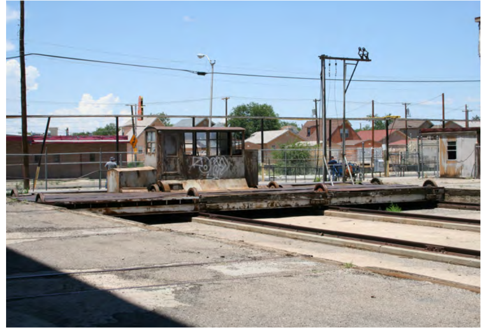
Transfer Table, west elevation.
