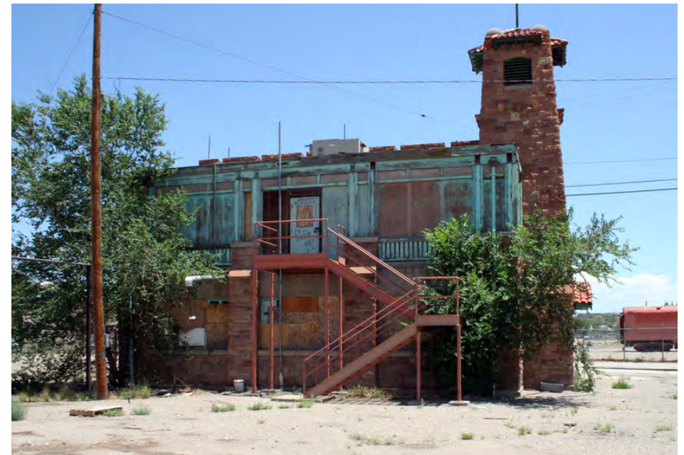
Firehouse, west elevation.
