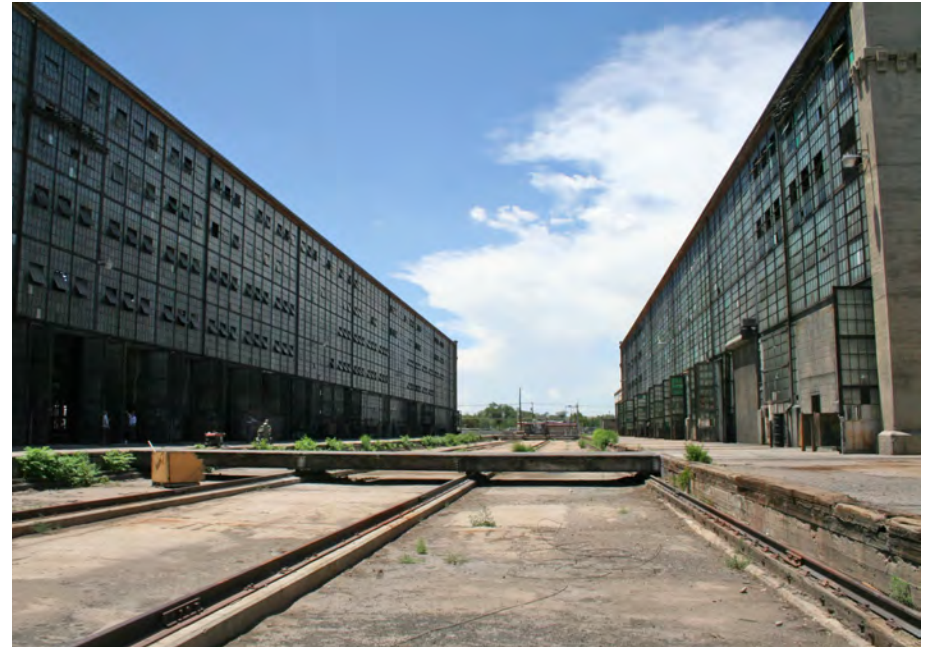
Transfer Table, view from the east side.
