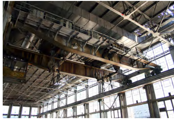
Boiler Shop, cranes in erecting bay.
