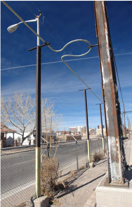
Perimeter street lighting and welding lines.
