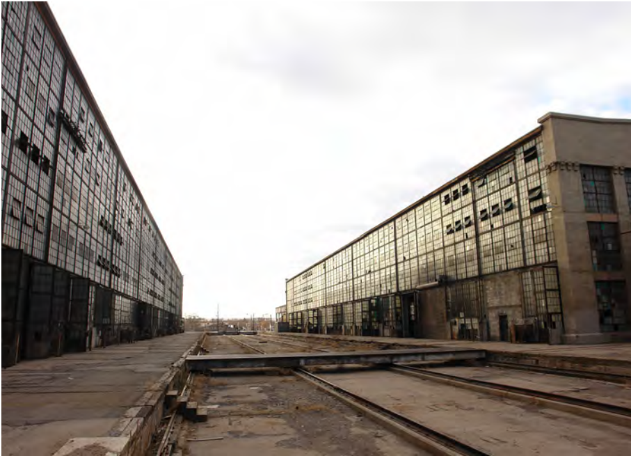
Transfer Table, view from east side.
