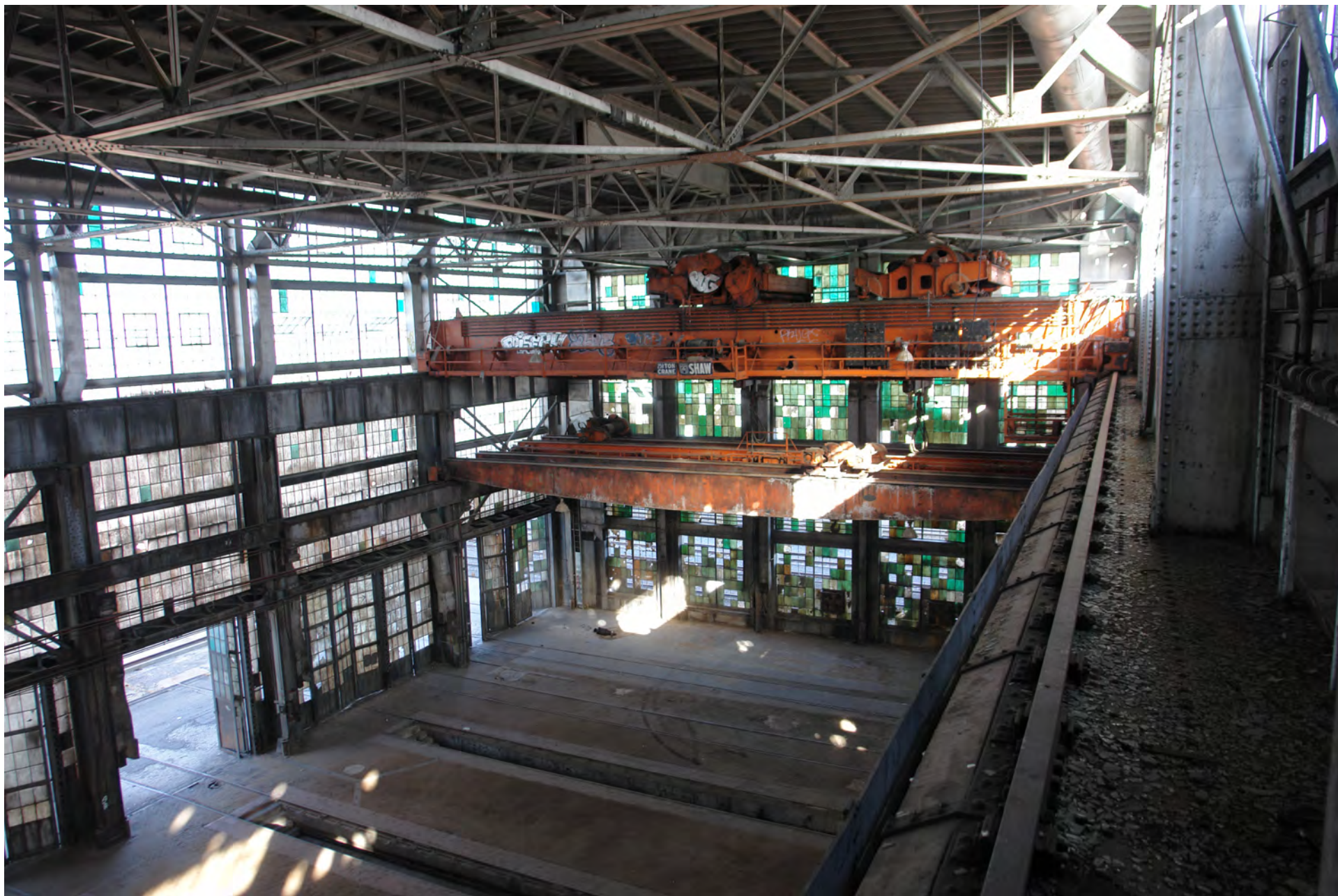
Machine Shop (2014), View from roof clerestory looking east.
