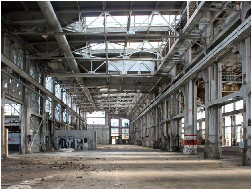
Boiler Shop, heavy equipment bay, pyramidal skylights
