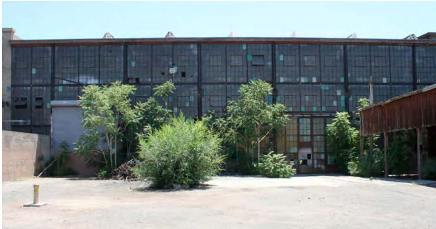
North elevation, exterior courtyard in foreground.
