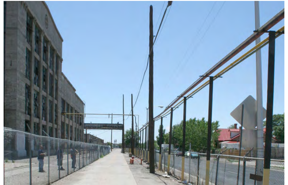
View south down fire runway between Machine Shop and Barelas neighborhood to the west.
