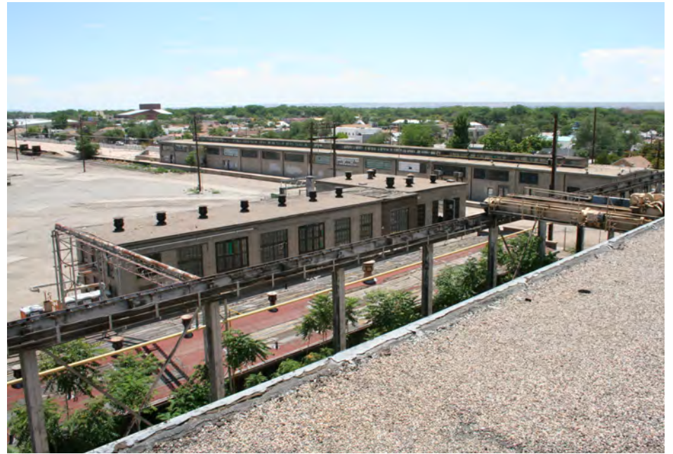
Storehouse, view from roof of the Machine Shop.
