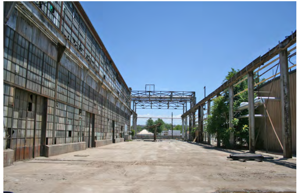
Bridge crane, view from west elevation.
