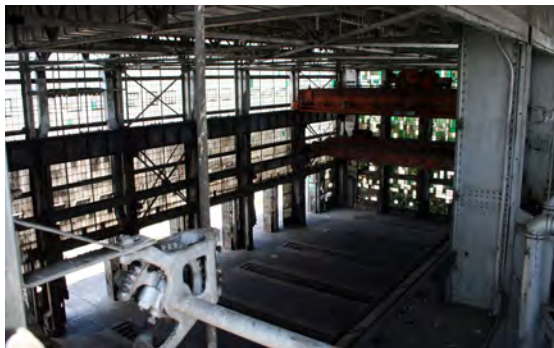
View of erecting bay from roof clerestory.
