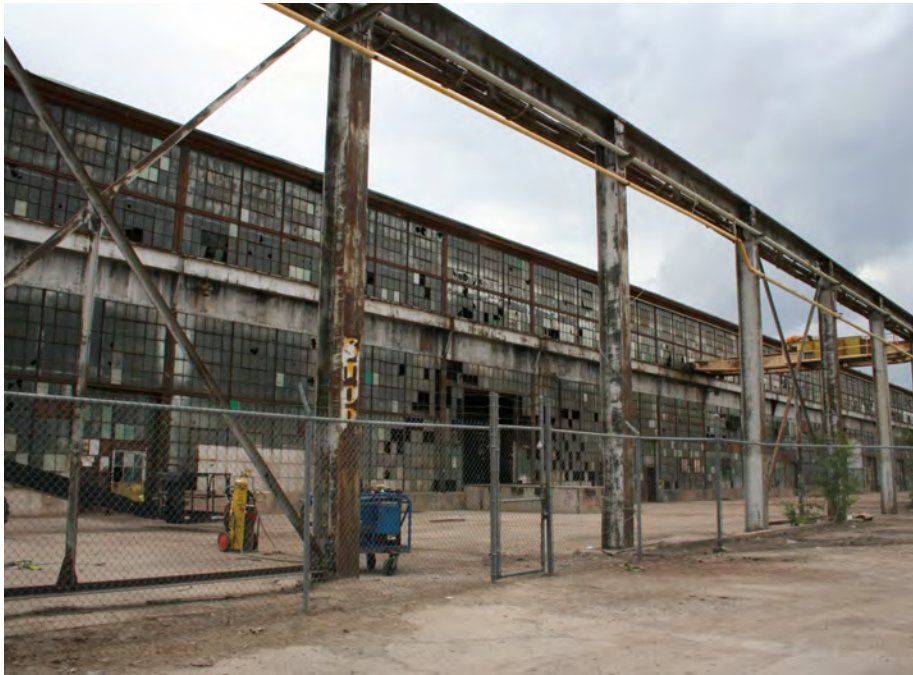
Bridge crane, view from southwest corner.
