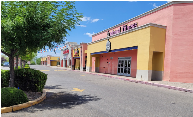
Vacant buildings at the Gateway Center at Menaul and Carlisle Boulevards.
