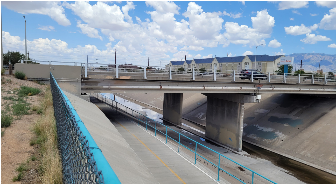
North Diversion Channel Multi-Use Trail.
