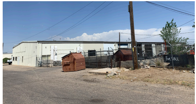
Substandard street conditions on the north side of Los Arboles Avenue toward Vassar Drive.
