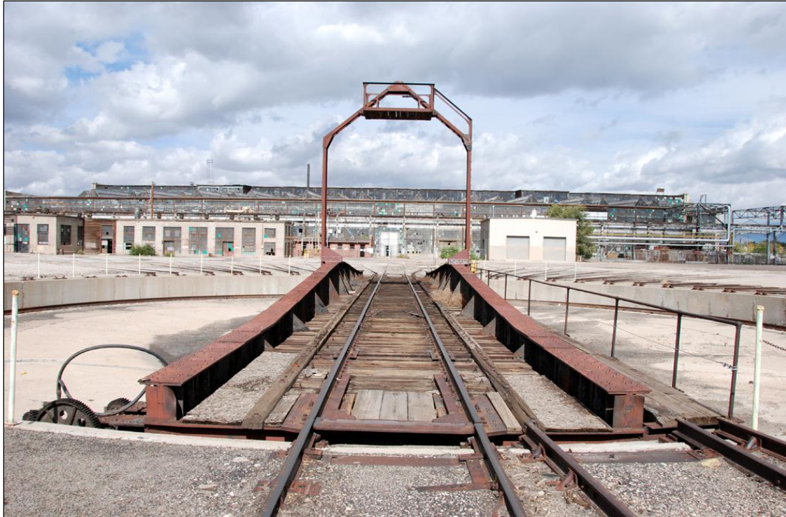
Figure 15 Working Rail Yards turntable with vacant Erecting/Machine Shop in the background
