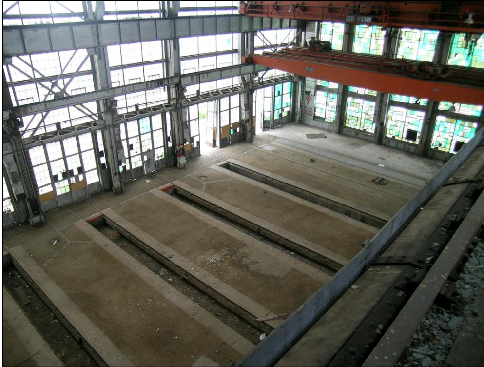
Figure 2 Vacant Erecting Shop Today – Note Intact 250 Ton Overhead Crane
