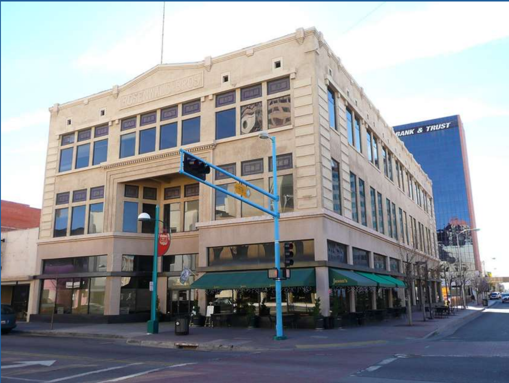
Rosenwald Building 320 Central Avenue SW, Albuquerque, NM 87102
