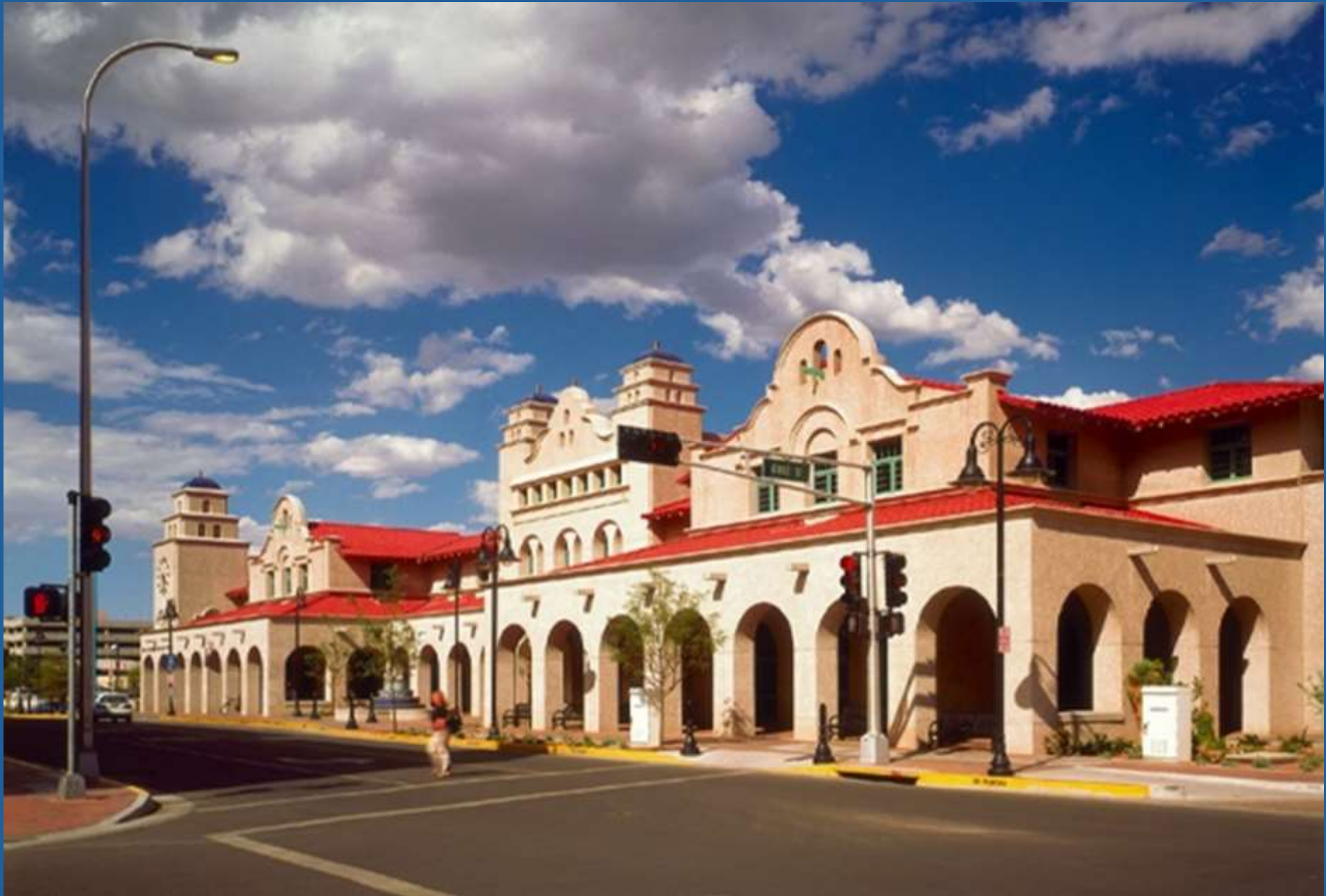
Alvarado Transportation Center 100 First St. S.W., Albuquerque, NM 87102
