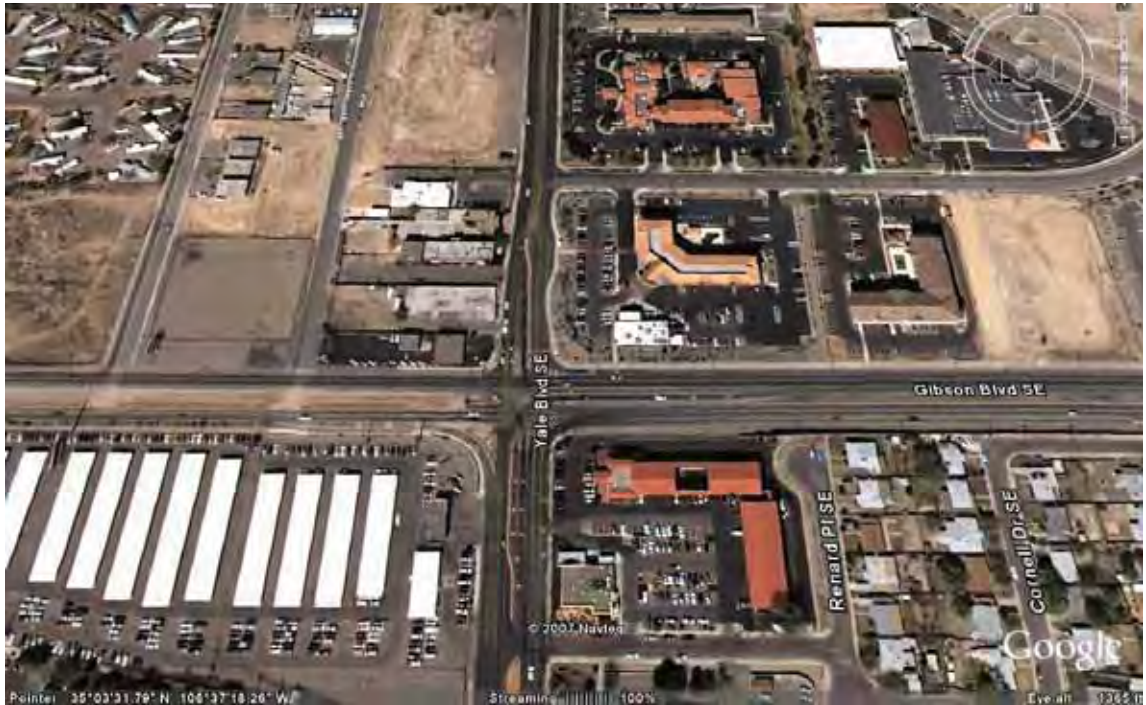
View of South Yale Boulevard and Gibson looking north. This intersection includes numerous hotels, restaurants and parking lots geared for the International Sunport. Note the existing mobile home park in the top left of photo.
